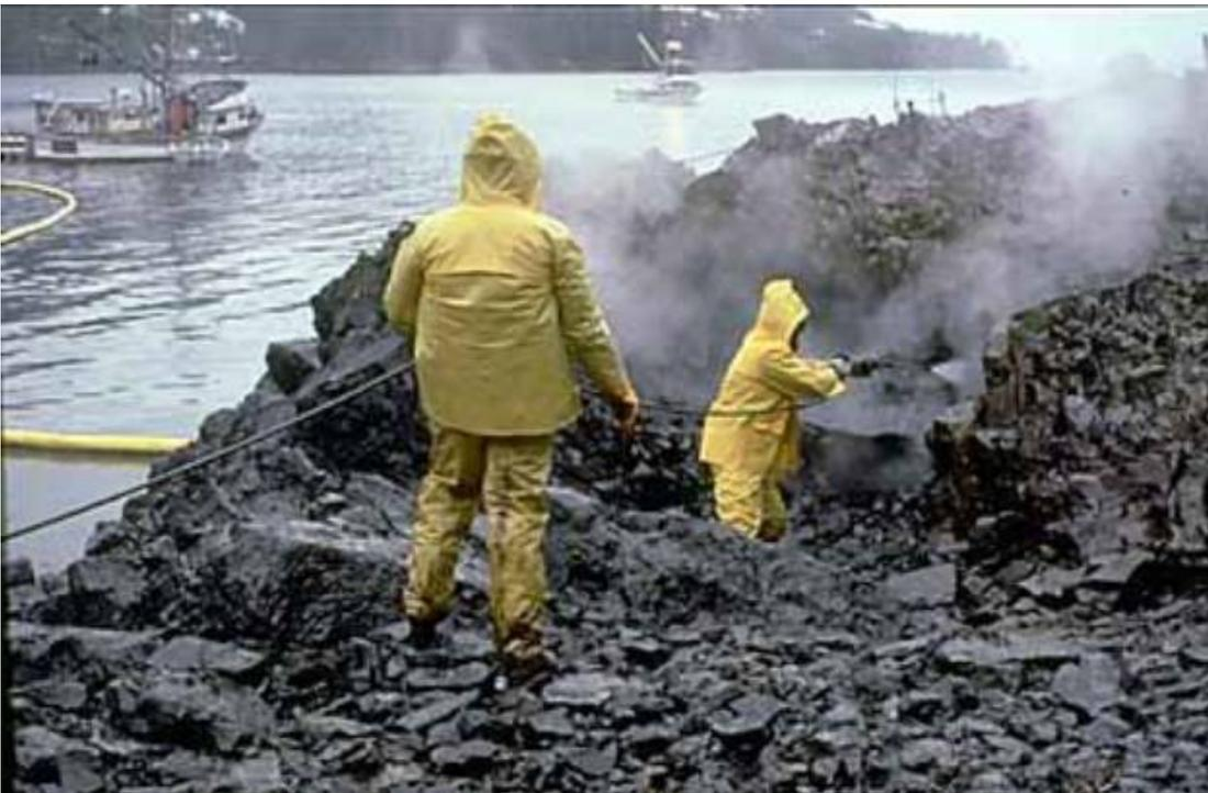
A brown sediment plume and sheens of refloat oil drift away from this oiled beach as it is cleaned by a team applying high-pressure, hot-water washing. Refloating of oil and release of sediment are often unavoidable consequences of shoreline cleanup that can cause additional environmental harm.
