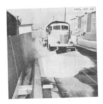
Fig. 2.11 Second Flushing Pass at Curb Using Three Nozzles.
