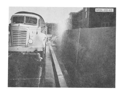
Fig. 2.12 Flushing Contaminant From Side Splash Boards into Drain Ditch Before Taking Radiation Reading on Test Surface.
