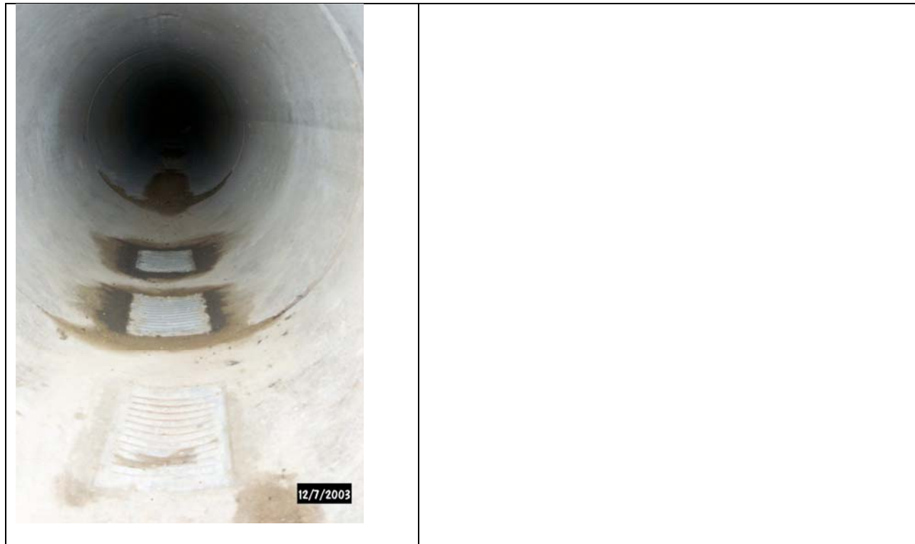
Figure 10. Recent bed load sampling in a residential area, Madison, WI (R. Bannerman, personal communication).
