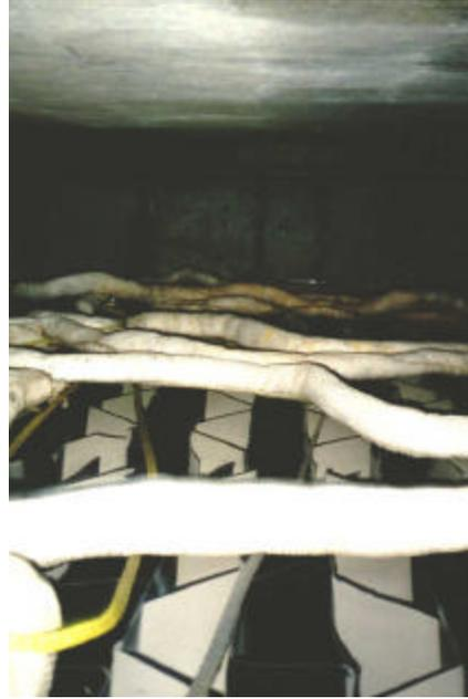
Inclined tube settlers and sorbent socks at MCTT installation in Milwaukee, WI
