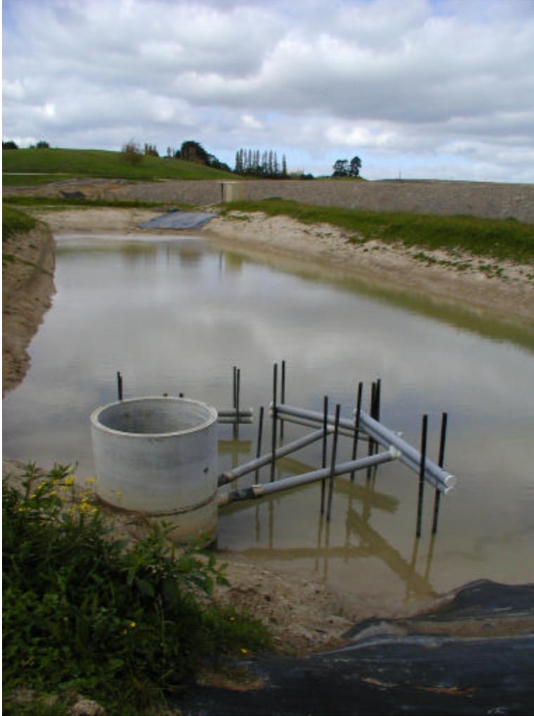
**Figure 21. Multi-level, perforated, floating discharges (decants) to better retain floc.**
