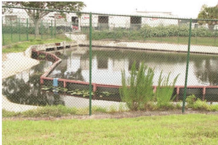
Orlando, FL, settling ponds to remove floc after alum injection, before discharge to lake
