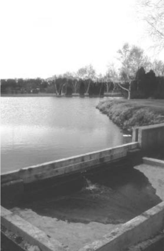
Adjustable spillway using boards in grooved weir
