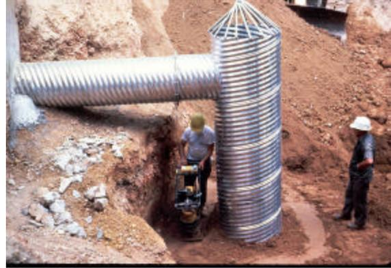
Vertical riser with safety bars, but culvert outlet should normally be placed near pond bottom to allow drainage for maintenance (State of Maryland photo)
