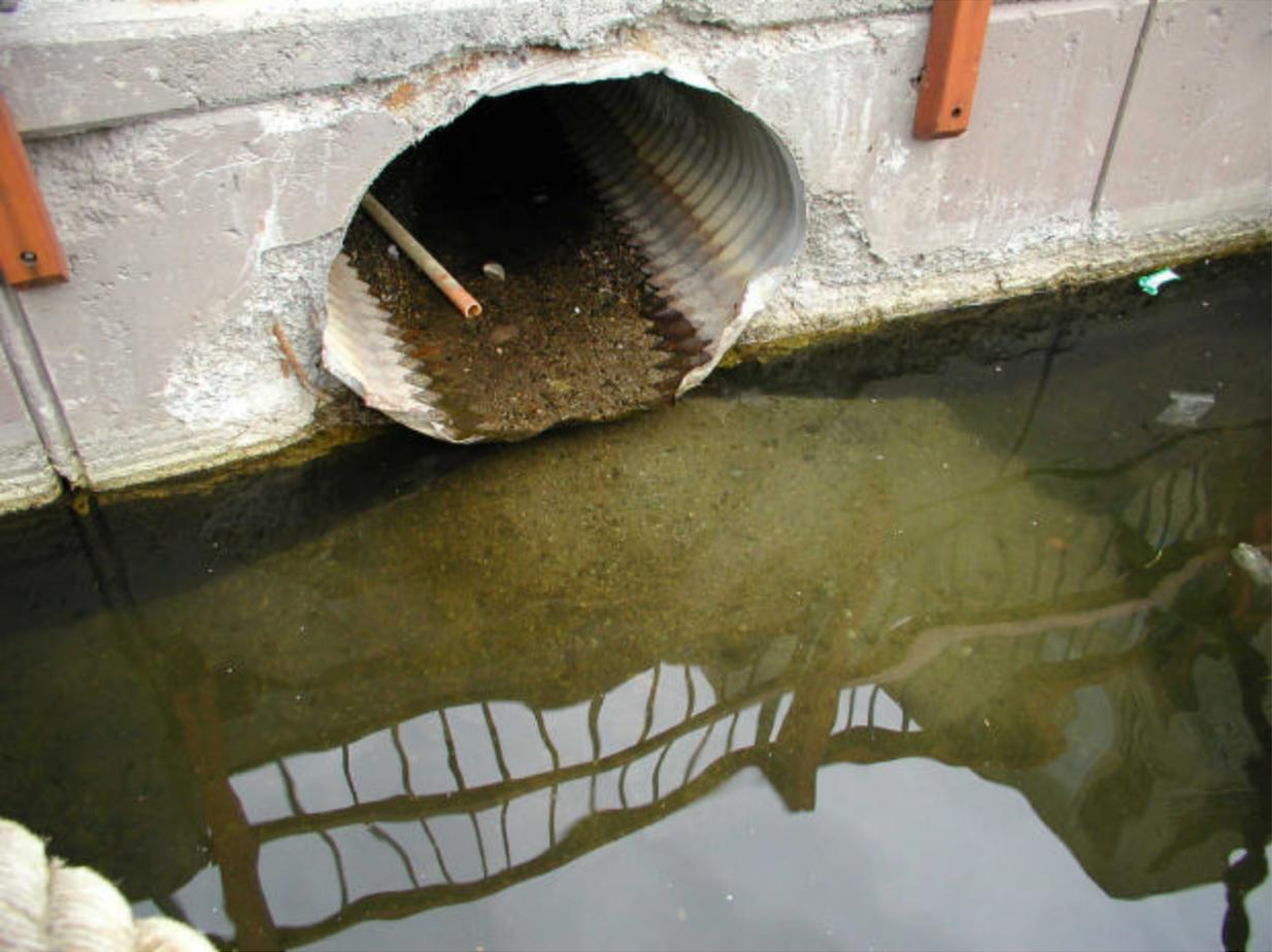
**Figure 65. Bedload sediment accumulation in sewerage and near outlet in pond (Snowmass, CO).**
