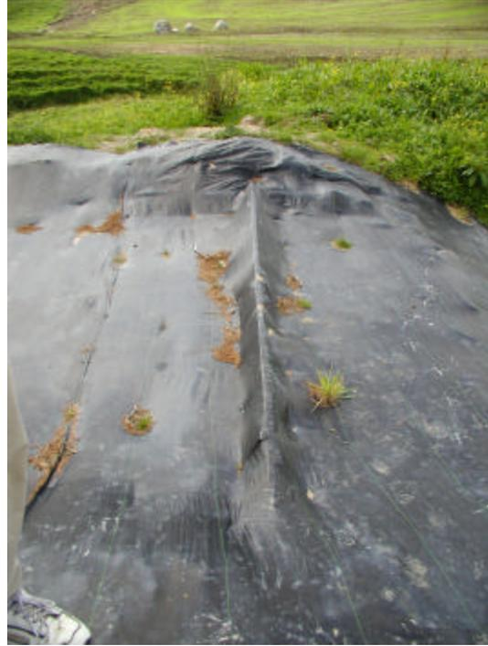
Temporary outlet control at construction site pond using a plastic membrane over a timber weir, Auckland, NZ
