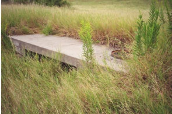
Box outlet emergency spillway at Gulf Port, MS, pond
