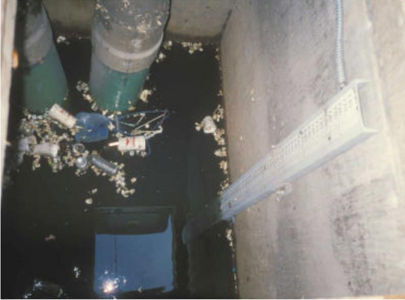
Figure 22. Oil and grease trap before downtown detention pond in Austin, TX.
