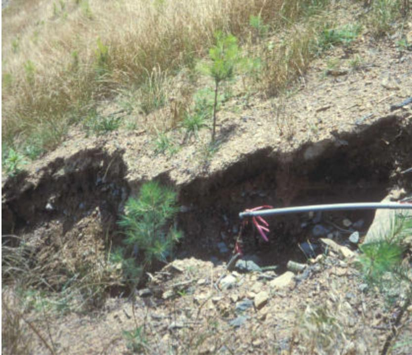
**Figure 28. Slope erosion due to seepage through pond dam.**
