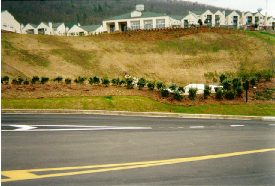
Figure 124. Emergency spillway flowing directly onto Bowling Drive.
