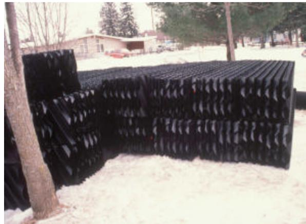
Inclined-tube settlers at Minocqua, WI, MCTT
