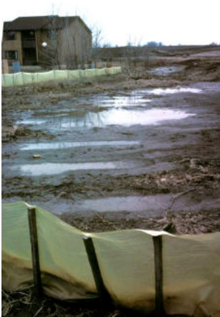
Middleton, WI, pond (heavy erosion filled pond)
