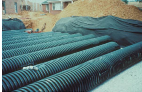
Underground plastic pipe detention facility during construction
