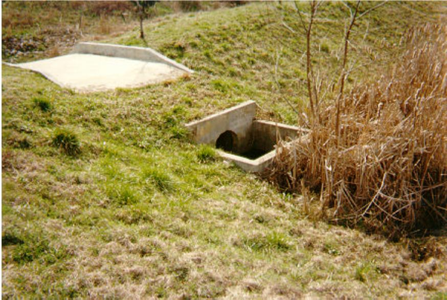
**Figure 115. Outlet structure, showing cattails partially blocking the 22 in orifices through concrete wall.**
