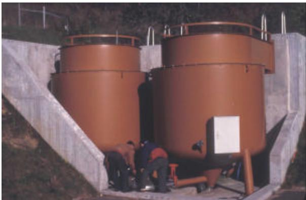
Gravity separation of wet weather solids in CSO swirl concentrators at Tangen, Germany
