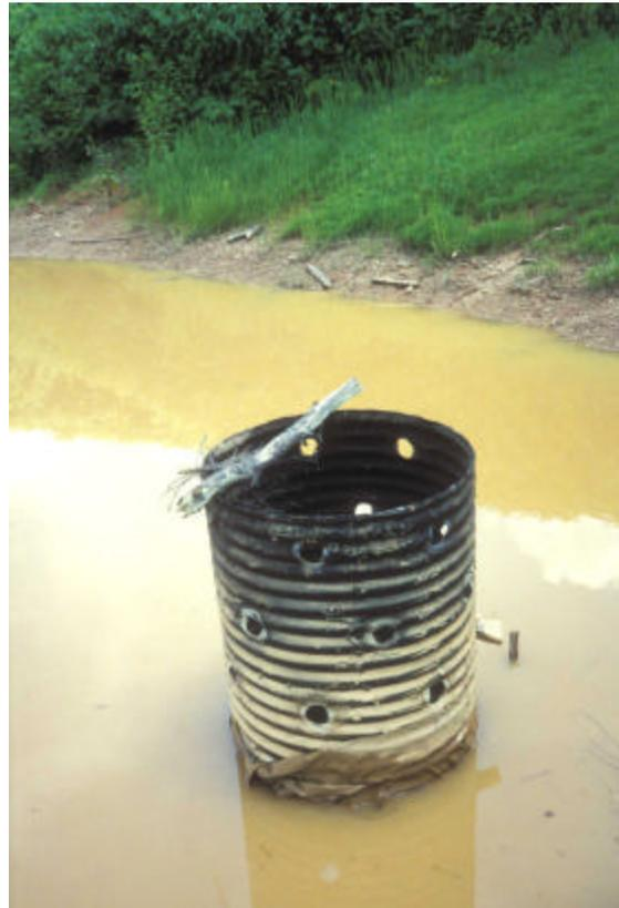
Typical perforated riser vertical stand-pipe at temporary pond, with no bar screens
