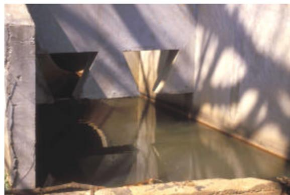
Slot energy dissipators at pond outlet
