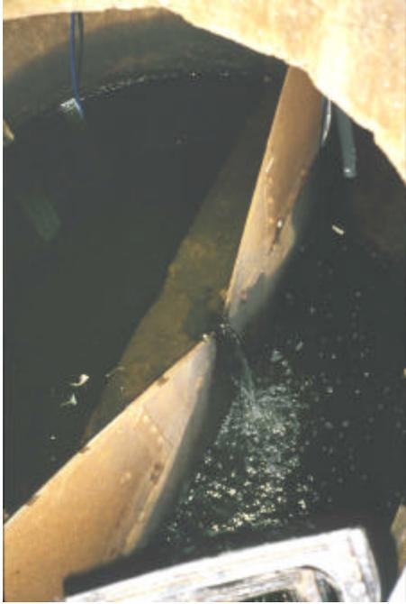
Retro-fitted v-notch weir in place of large rectangular weir at Monroe St. pond in Madison, WI
