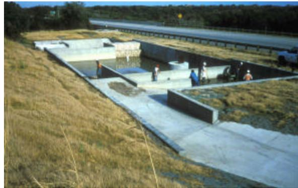
Austin, TX, MoPac Highway treatment unit using accident discharge diversion capture pond, dry pond, and horizontal flow sand filter
