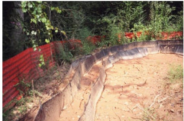
**Figure 138. Filter fence installations showing areas of sedimentation where water pools behind the fences**
