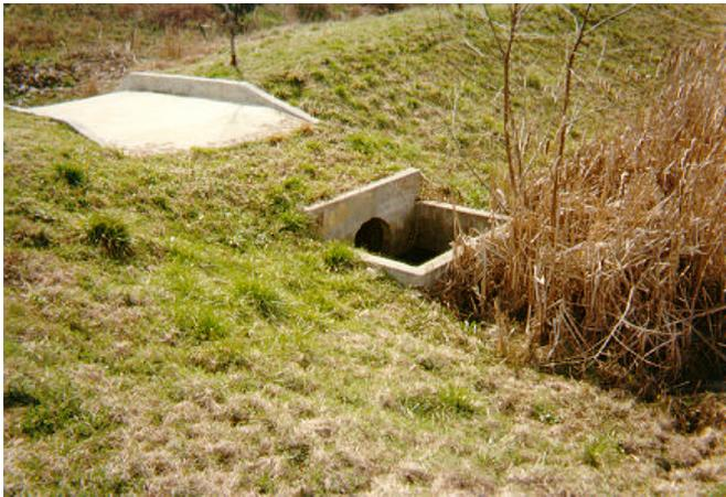
Birmingham, AL pond outlet structure, showing cattails partially blocking 22 in orifices through concrete wall (John Easton photo)
