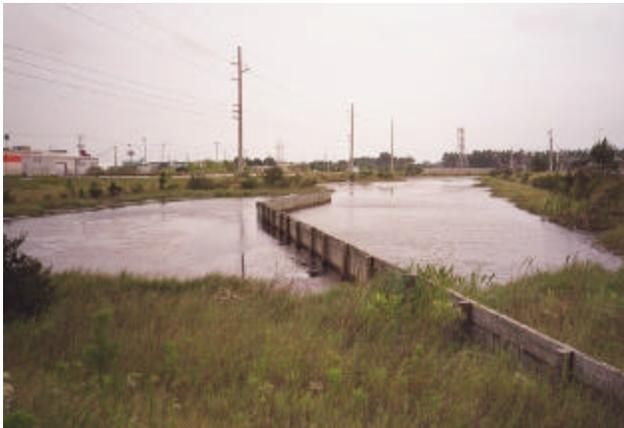
Baffle fence constructed in pond to separate inlet (to right) from pond outlet (to left), forcing water to travel further down pond length.
