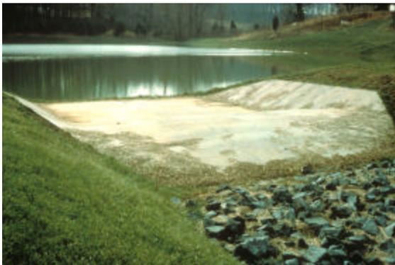
Large concrete emergency spillway
