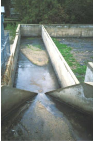
Sedimentation forebay before vertical flow sand filter at Austin, TX
