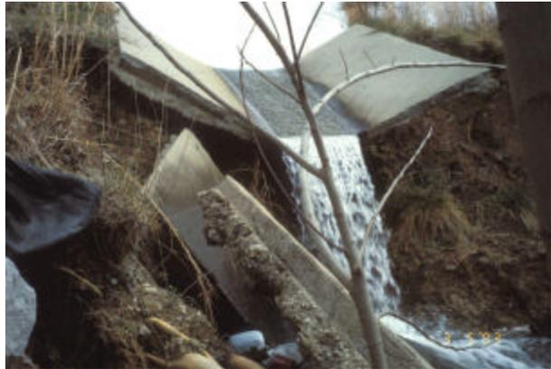
Broken concrete spillway due to undercutting (photo by Mark Burford)
