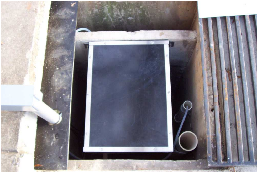
Figure 5. Prototype UpFlo™ filter shown along with inlet grate cover
