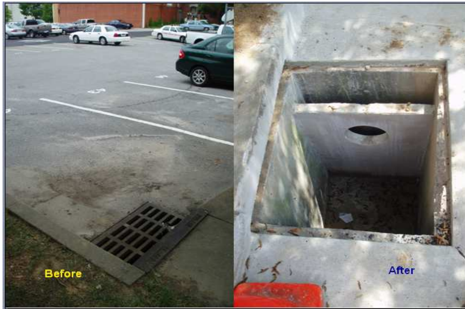
Figure 4. Inlet before and after modifications
