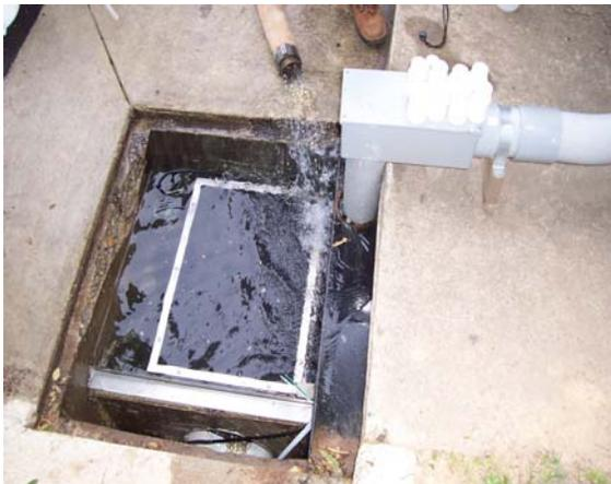
**Figure 4-5: Steady state filtration rate at the height of the bypass weir**
