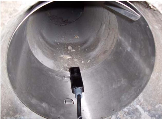
Figure 4-20: Area-velocity sensor installed in effluent pipe.
