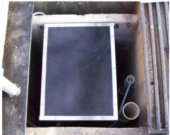
Figure 4-23: Installed prototype Up-Flo™ Filter (no media) with sampling and monitoring lines
