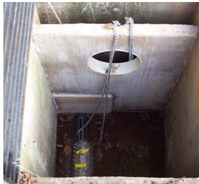
**Figure 4-25: YSI Sondes installed in sump (another is behind baffle wall for effluent)**
