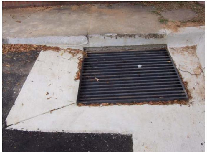
**Figure 3-7: Completed modified inlet with new inlet grating.**
