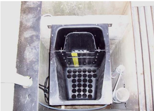
Figure 4-22: Prototype Up-Flo™ Filter and sampling gear installed in catch basin.
