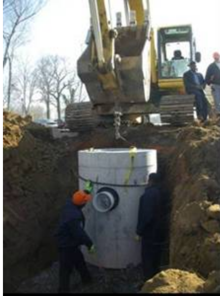
Figure 1.3 Installation of Tuscaloosa Up-Flo Filter.
