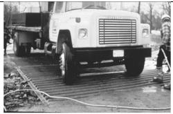
Truck being cleaned as it leaves construction site for public right-of-way.
