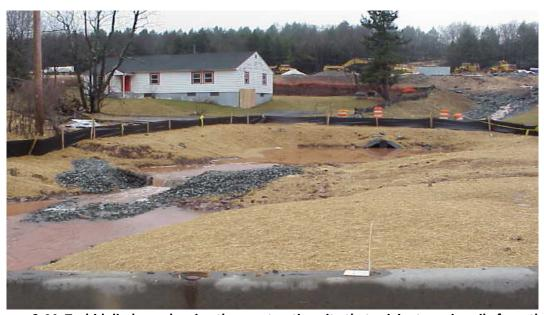
Figure 6-44. Turbid discharge leaving the construction site that originates primarily from the flow from the waste area but also with intervening site area (D. Lake photo)
