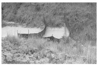
Figure 6-92. Silt fence check dams on a construction site (practice not commonly approved; silt fences best use for sheet flows). Jamie Lyles; UA student.
