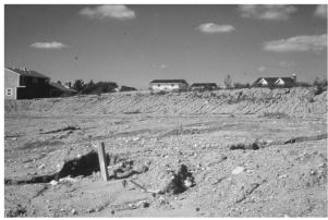
Figure 1-31. Unattended severely eroded land causes great amounts of sediment loss and requires site regrading.
