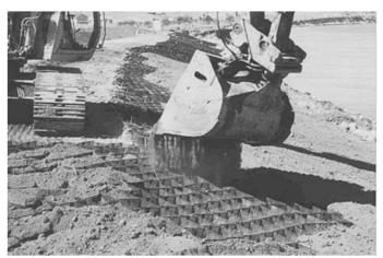
Figure 5-6. Geogrids being filled with sand for bank protection (IECA photo)
