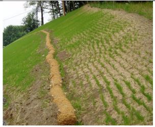
Slope stabilization using tracking, seeds and mulch, with coir logs (D. Lake photo)
