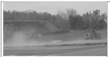
Fugitive dust losses and traffic safety problem as heavy equipment was being driven on unprotected construction roads near existing roads during period of high winds.
