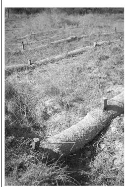
Coir (cocoanut fiber) rolls/logs and soil adhesives for slope stabilization project at Newport Beach, CA, wildlife refuge.
