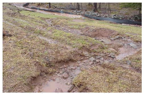
Figure 6-42. West sediment basin in the waste area with an eroded cut in the downstream face of the dam (D. Lake photo)
