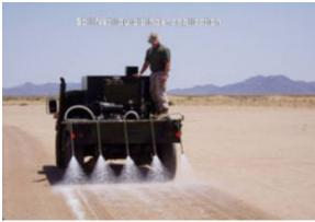
Figure 5-71. Applying polymers to soil (Source: <a href="http://www.soilnetllc.com/dust.html">http://www.soilnetllc.com/dust.html</a>).
