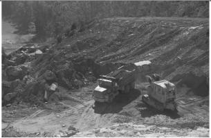
Continuous operations at a solid waste landfill require special precautions to prevent excessive erosion. This site has a large sediment pond, with pre-treatment forebays, plus a final sand filter, to meet their 50 NTU discharge permit requirement for turbidity.
