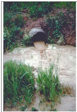
Culverts can be haphazardly installed during construction operations. They can provide high energy supercritical velocities at their outlets that need to be reduced to prevent scour.
