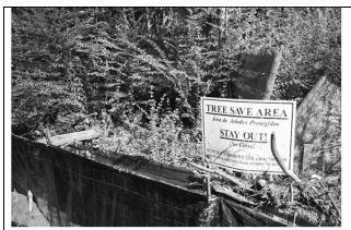
Barrier fencing setting outer limits of disturbance at construction site.
