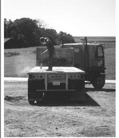
Vehicle being cleaned as it leaves a construction site to prevent debris from affecting pubic roads.
