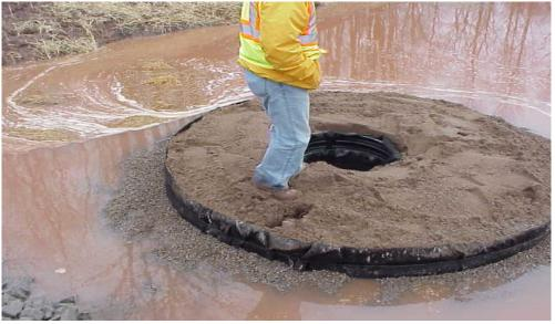
Figure 6-46. A sand filter constructed around a vertical dewatering riser in a sediment basin within the project site (D. Lake photo)
