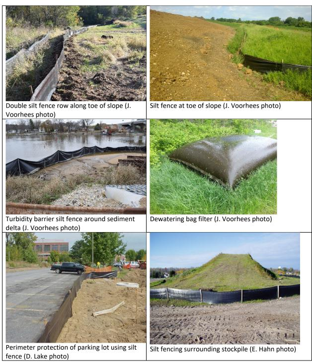
Figure 6-83. Uses of filter fabric material and silt fences at construction sites.
