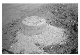
Figure 2-15. Proprietary filter fabric storm drain inlet covers
