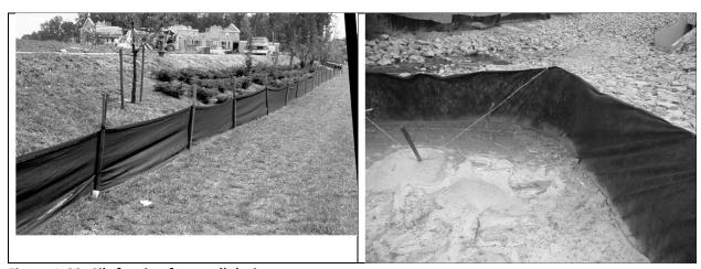
Figure 1-32. Silt fencing for small drainage areas
