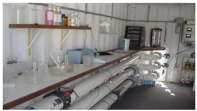
Figure 6-80. This is the inside of the control center for the polymer operation. Constant monitoring of the NTU levels is provided by the continuous turbidity meters on the back wall (D. Lake photo)
