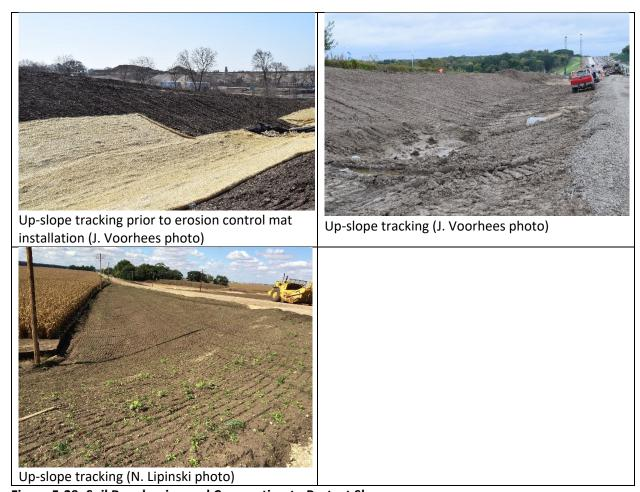
Figure 5-39. Soil Roughening and Compaction to Protect Slope
