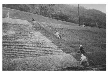
Figure 5-48. Installation of Netting over Mulch
