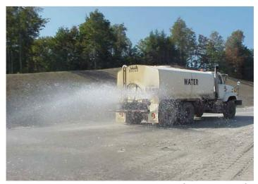
Figure 2-9. Dust control with water truck (D. Lake photo)
