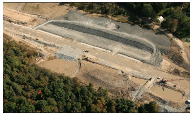
Figure 6-81. This aerial view shows the erosion and sediment control system just north of Scoby Road located at the right of the photo. Note the plastic lined swales. Flow is from left to right as it works from a swale through a pipe to the linear sediment trap, the small basin with a pipe to the larger basin where the polymer system is located. The shale buttressing for slope stability and drainage is prominent in the upper portion of this part of the project (NYS DOT photo)
