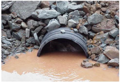
Figure 6-43. The western sediment basin outlet pipe. There is no reduction in turbidity due to flow through joints that have been separated by riser damage from winter ice action (D. Lake photo)
