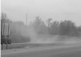
Another example of fugitive dust causing potential traffic safety problems. Construction was halted this day due to high winds at this road-widening project, but unstabilized and exposed ground still allowed excessive dust losses.
