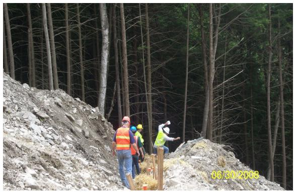
Figure 5-54. Remediation work on the Millennium slope above Peas Eddy to control and dissipate runoff. (NYSDEC photo)
