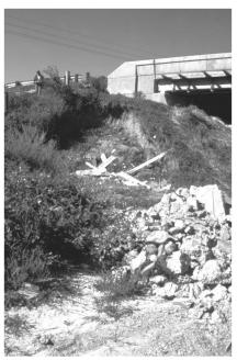
Figure 1-30. The lack of an appropriate diversion structure to safely drain water down sensitive slopes can cause much damage and sediment loss.
