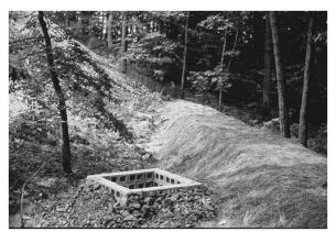
Figure 2-14. Cinder block and gravel barrier to protect inlet (SCS photo)
