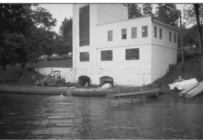
These two photos at the New York State Electric & Gas Corporation hydroelectric plant on Keuka Lake demonstrate the use of water structures as cofferdams. Two tubes of polyethylene wrapped with a geotextile are filled with water to act as a low ground pressure, environmentally friendly cofferdam. They can be installed and removed quickly.
