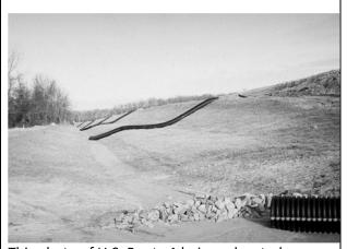
This photo of U.S. Route 1 being relocated around Dover, Delaware shows pipe slope drains that carry sediment laden runoff downslope to a collector swale. Note that the side slopes are graded and seeded as the work progresses to keep soil from washing down.
