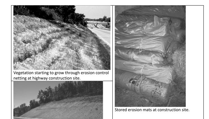
Newly installed erosion control mats on steep highway embankment.
