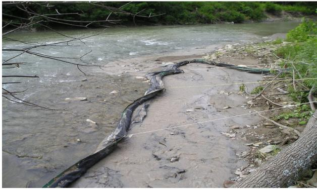
Figure 6-73. Turbid discharge is shown here entering Cattaraugus Creek at the Scoby Road outlet approximately 400 feet to the west and down slope of the project limits (D. Lake photo)
