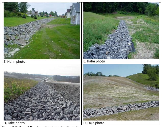
Figure 5-3. Gravel lined swales at construction sites
