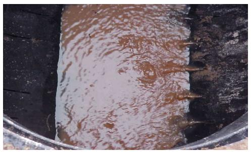
Figure 6-47. Turbid flow moving through the sand filter system, entering the perforated outlet pipe which discharges to a drainage swale offsite (D. Lake photo)
