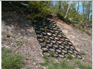
Bio-technical slope protection on Whiteface Mtn. (NY) using old ski lift rubber bushings (D. Lake photo)
