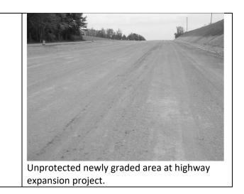
Figure 1-23. Minimize Exposed Soil
