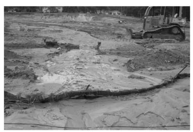
Figure 6-98. Overloaded silt fence. Caroline Sandel, UA student.
