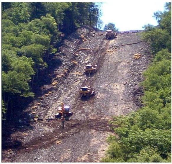
Figure 5-53. Slope repair work being done on the very steep slope. Note that the four pieces of equipment are tethered together with steel cables (Binghamton Press photo)
