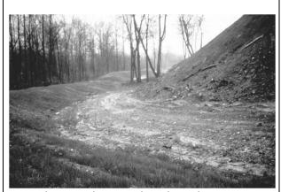
Large diversion berm and swale to divert water from downslope area at an abandoned mine site (SCS photo).
