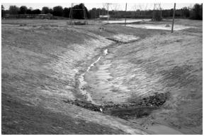
Figure 1-16. This exposed site is under a state shutdown order for destroying 2 acres of walleye spawning area in a nearby lake. 65 acres of the 70 acre site was stripped exposing soil containing 75 – 98 percent fines that could not settle out on site.
