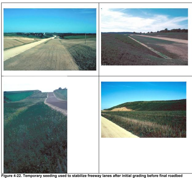
Figure 4-22. Temporary seeding used to stabilize freeway lanes after initial grading before final roadbed construction.
