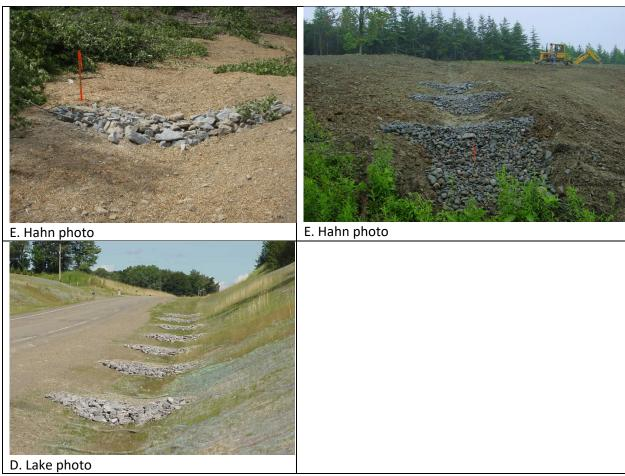
Figure 5-30. Well-constructed rock check dams.
