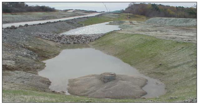
Figure 6-79. This system of two sediment traps south of Scoby Road had two different outlet types. Together they limited the discharge to 25NTU (D. Lake photo)
