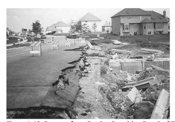
Figure 1-10. Damage from Erosion Requiring Repairs (IECA photo)
