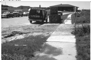
Excessive tracking due to insufficient or non-maintained graveled access needs to be corrected.
