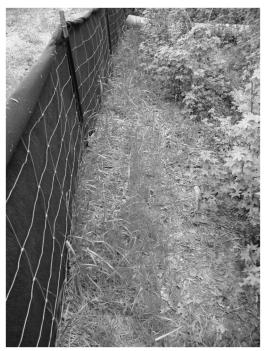
Figure 2-2. Downslope side of perimeter wire-backed silt fence intercepting sheetflows.
