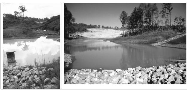
Figure 1-33. Sediment ponds for larger construction areas
