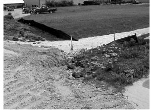
Same site as prior photo showing sediment load overtopping silt fabric fence due to lack of maintenance (J. Voorhees photo)
