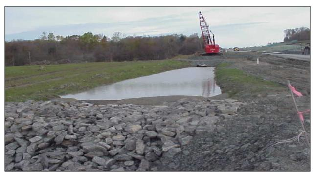
Figure 6-78. This linear sediment trap is located north of Scoby road upstream from a sediment pond. Its pea gravel/rock dam outlet reduced the sediment load from 2,600 NTU to 40 NTU. Constant maintenance was required (D. Lake photo)
