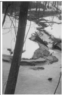
Filter fabrics rarely made adequate check dams
