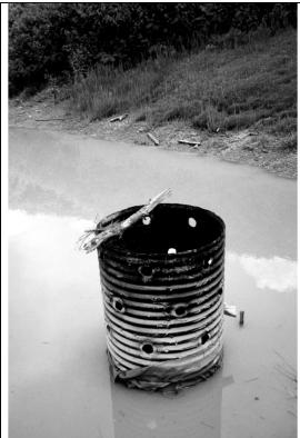
Vertical riser having multiple outlets and wrapped with geotextile fabric
