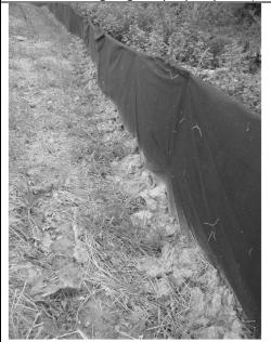
Well-installed filter fabric silt fence, with bottom of fabric buried and backfilled to prevent underflow of sediment
