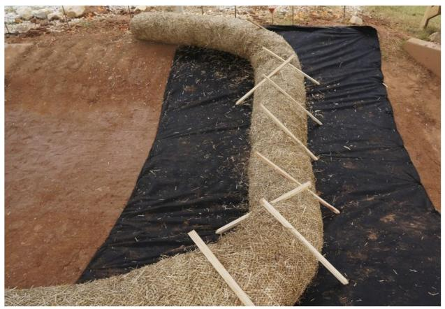
Figure 5-35. Coir log check dam placement.
