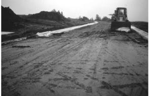
End of season construction site shutdowns can also result in excessive erosion during late winter and early spring rains during periodic thaws unless the site is well-stabilized for the season.
