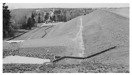
Figure 5-50. Slope drains on terraces (Source: Tobiason, et al. 2000)
