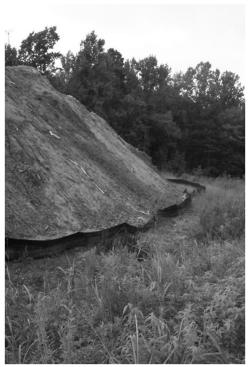
Figure 6-97. Use of silt fences around storage pile. Caroline Sandel, UA student.
