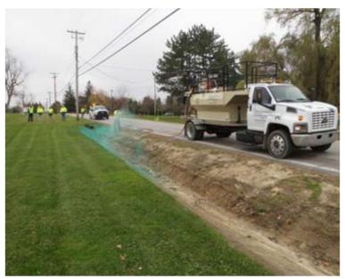
Figure 5-72. Applying hydromulch mixture to channel (Source: http://www.crwp.org/files/RD\_Mulch\_FactSheet\_July2012.pdf).
