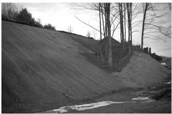
Figure 5-49. Various Slope Protection Treatments and Tree Conservation
