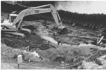
These photos show the use of a Port-A-Dam system in use at Nuclear Lake in Dutchess County, New York. This 54 acre lake is about 12 feet deep and would have had to be pumped dry to fix the dam. This system was installed by divers, then the interior pumped dry for working, protecting lake ecosystem.
