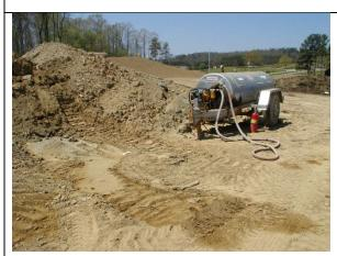
Fuel spillage at re-fueling area is both hazardous and damaging.
