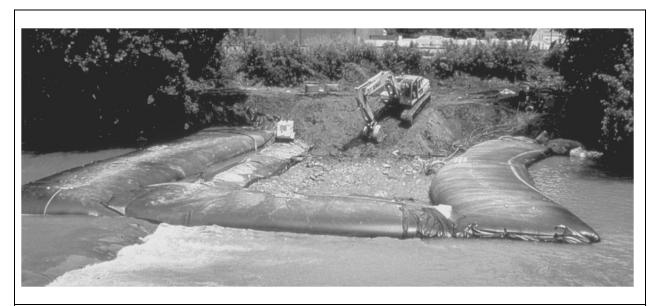
This is another example of how utility line crossings can be accomplished without routing construction equipment through the stream. This Aqua-Barrier allows one side to be completed then the set up can be moved to the opposite bank for completion of the crossing.
