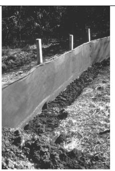
Layer of silt captured against bottom edge of newly installed silt fabric fence
