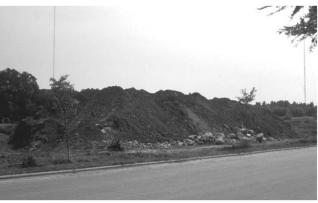
Figure 2-19. Soil stockpile next to road needing protection
