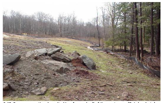
Figure 6-40. Excess excavation deposited in a forward cell of the waste area (D. Lake photo)
