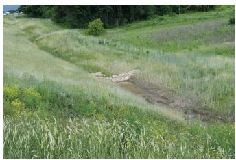
Figure 5-32. Check dam in new channel at construction site with mature grass (J. Voorhees phot
