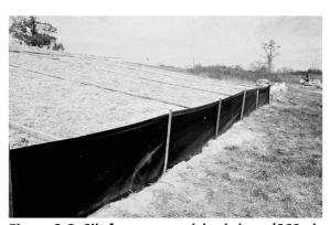
Figure 2-3. Silt fence on mulched slope (SCS photo).
