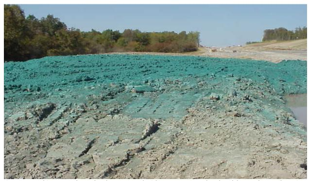
Figure 6-77. This exposed area has been treated with temporary seed and mulch to reduce soil erosion losses (D. Lake photo)
