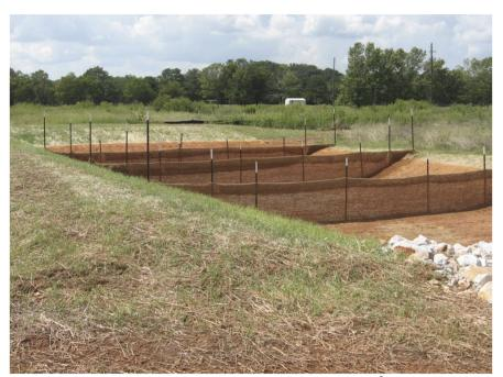
Figure 6-33. Example of porous baffle made of 700 g/m<sup>2</sup> coir erosion blanket as viewed from the inlet
