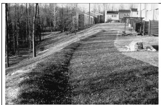
A small berm and sodded swale divert flows from newly graded and mulched hillside.
