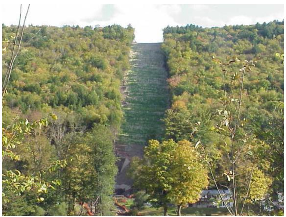
Figure 5-55. Peas Eddy slope stabilized with slope breakers and seeding with a double layer of jute mesh over straw mulch over the entire slope face (D. Lake photo)
