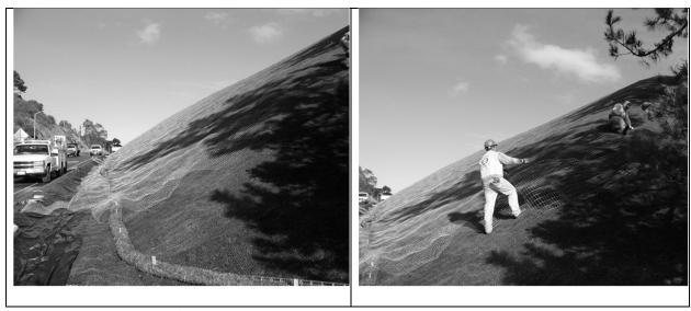
Figure 5-47. Installation of Wire Netting over Mulch
