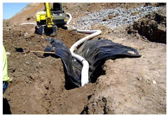
Figure 5-60. Placing a filter wrapped perforated drain pipe in the slope (Abscope Construction photo)
