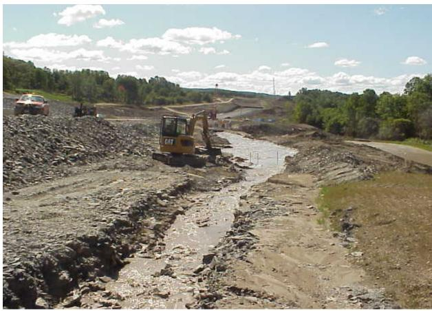
Figure 6-72. Groundwater is flowing in the drainage ditch along the west side of the construction area towards Scoby Road. The flow rate from this source was a fairly constant 130 gallons per minute (D. Lake photo)
