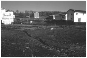
Large-scale sheet and rill erosion and isolated gully erosion beginning to start at an inadequately protected construction site.
