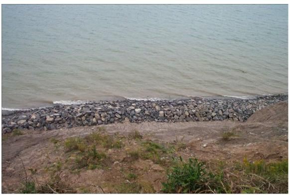
Figure 5-58. On-shore toe revetment at the bottom of the Lake Bluff slope to resist wave action (T. Cassel photo)
