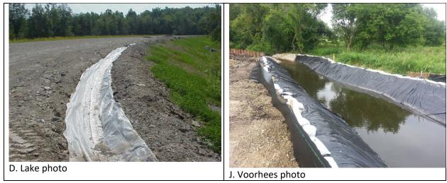
Figure 5-2. Lined temporary bypass channels at construction sites
