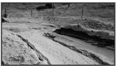
Figure 6-51. Pond inlet channel full of sediment and buried floc blocks (Source: Beca Carter Hollings & Ferner Ltd, undated)
