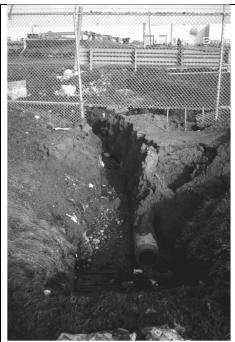
Poor grading directed runoff away from drain inlet and to the unprotected slope. Expensive repairs are now needed.
