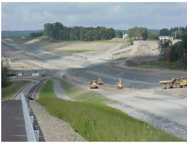
Figure 6-82. Final grading for the pavement base layer is almost completed in the Scoby Road segment (D. Lake photo)
