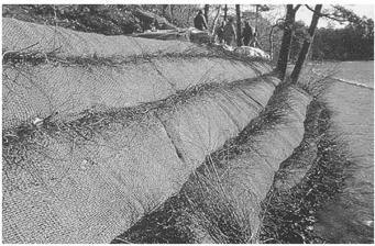
Figure 5-5. Bioengineered channel slopes (IECA photo)
