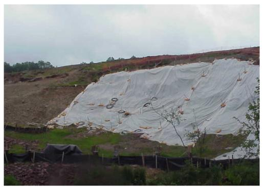
Figure 6-48. Steep slope at Parksville on-ramp construction covered with plastic to prevent erosion into the Little Beaver Kill (D. Lake photo)
