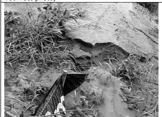
Inspections must require replacement of damaged erosion controls (J. Voorhees photo)
