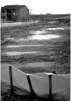
Figure 6-27. Temporary construction site pond filled with sediment
