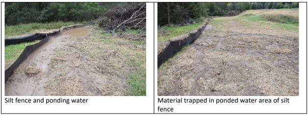
Figure 6-84. Silt fences accumulation of material (J. Voorhees photos)
