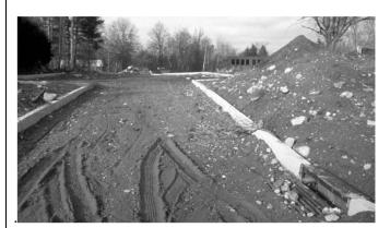
Control of runoff is critical at the beginning of construction. Here the stormwater infrastructure is in place but the 24 inch storm sewer is 75% plugged with sediment. Note the large size of the material on the catch basin grate.
