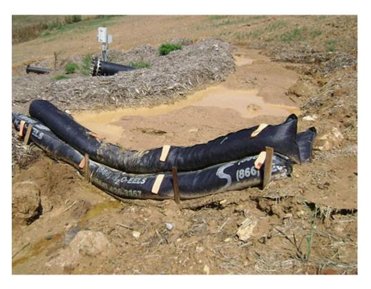
Figure 5-34. Wrapped check dams (Source: <a href="http://www.priceandcompany.com/prod-checkdams-erosioneel.html">http://www.priceandcompany.com/prod-checkdams-erosioneel.html</a>).
