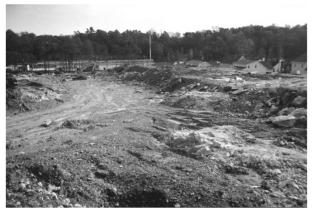
Figure 2-5. Large expanses of unprotected soils left exposed for long periods cause most of the sediment losses from construction sites.
