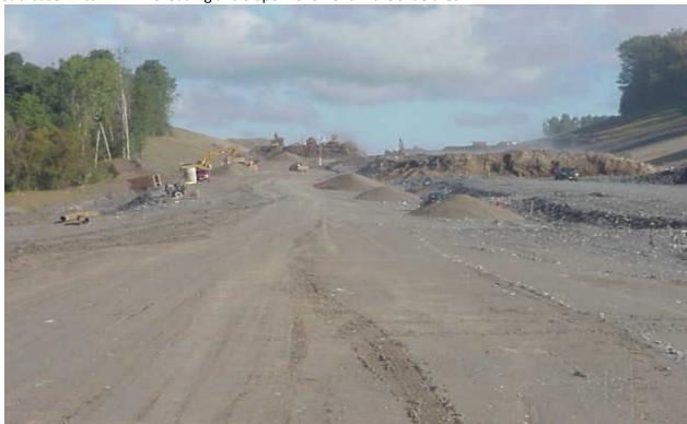
Figure 6-71. Construction equipment is removing previously placed embankment material to unload the slide area north of Scoby Road. Note that all runoff drains towards the foreground (D. Lake photo)
