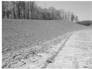
Roughened slope after compaction by Sheep's foot compactor.
