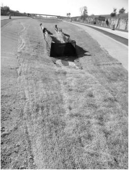
Inlet protected by filter fabric, thick matting to protect new grass, and chemically stabilized soil (Illinois).
