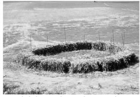
Straw bale barrier showing large gaps between bales and decomposing bales, needing replacement (SCS photo). Most agencies no longer allow the use of straw bale barriers.
