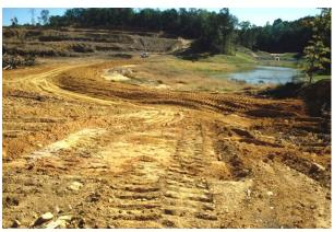
Figure 2-4. Sediment pond at landfill
