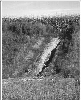
Another unfortunate example of poor grading allowing runoff to miss protected downslope channel.
