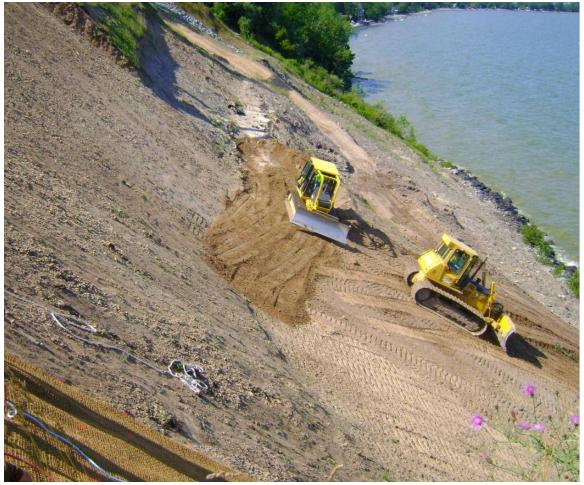
Figure 5-61. Finished grading on the slope. 2:1 on the lower slope and 1:1 on the upper slope. Note the jute mat on slope in foreground (Abscope Construction photo)
