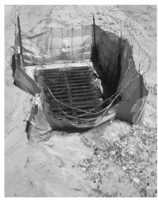
Large accumulation of debris surrounding filter fabric inlet barrier, requiring maintenance.
