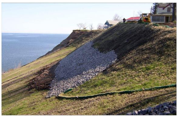
Figure 5-65. Slope drain and rill repair on Lake Bluff (T. Cassel photo)
