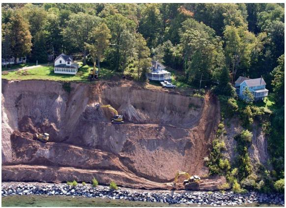
Figure 5-59. Slope construction taking place on Lake Bluff. Note the ramps for access to grade out the design slopes (T. Cassel photo)
