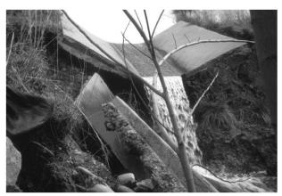
Figure 5-26. Broken concrete channel due to undercutting (photo by Mark Burford).
