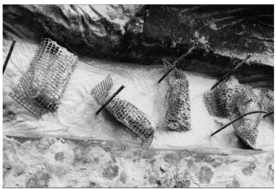
Figure 6-50. Floc blocks within channel between forebay and pond (Source: Beca Carter Hollings & Ferner Ltd, undated)
