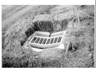
Typical straw bale barrier surrounding inlet (notice tight bales and large amount of sediment collected around outside of bales, needing removal). Most agencies no longer allow the use of straw bale barriers.
