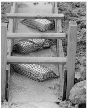
Figure 6-49. Floc blocks and flume detail, initial installation (Source: Beca Carter Hollings & Ferner Ltd, undated)
