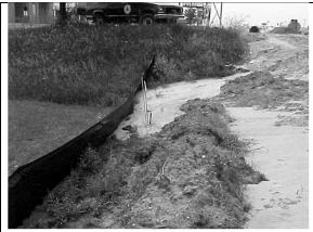
Large sediment load captured by silt fence, maximum load before needed maintenance (J. Voorhees photo)
