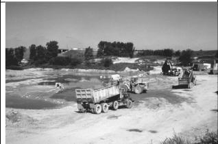
Temporary pond at highway construction site in area where hauling trucks are washed prior to reentering roads (WI)
