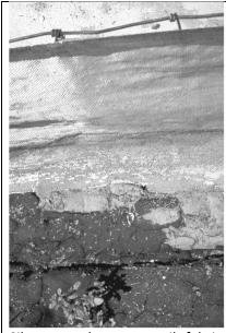
Silt captured on woven silt fabric
