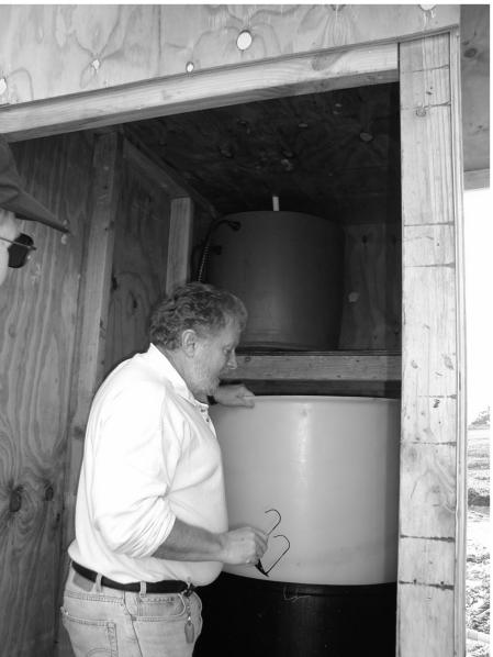
Figure 6-67. Earl Shaver, then of the Auckland Regional Council, showing the main components of the rainfall-driven chemical dosing system.
