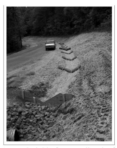
Figure 5-33. Fiber check dams (Source: McLaughlin, et al. 2009).
