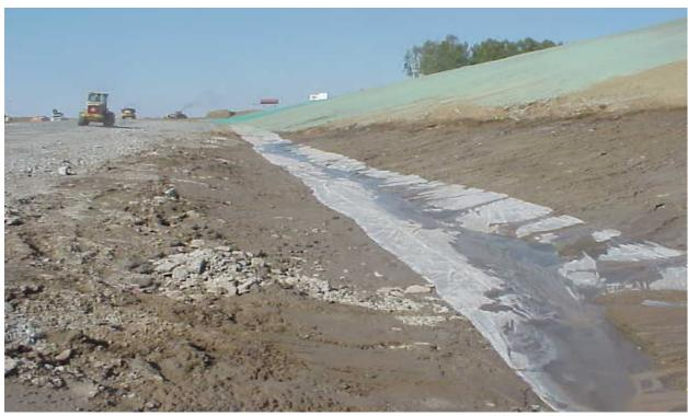
Figure 6-75. The plastic lined swale conveys groundwater through areas of fine grain soil limiting the erosion. Note the slope stabilization (D. Lake photo)
