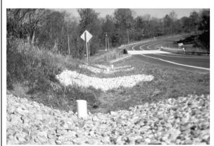
Series of riprap check dams spaced to cause ponding between dams (SCS photo)
