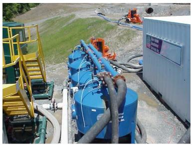
Figure 6-69. Sand filters for floc removal after liquid polymer treatment at construction site (D. Lake photo)
