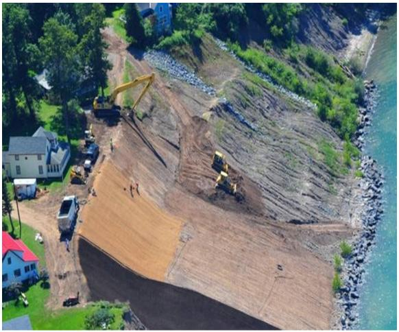
Figure 5-62. The sequencing of the slope construction can be seen in this photo. Rough grading and drainage installation has been completed with some still evident at the top of the picture. Finish grading is occurring in the middle while below that the jute matting is being placed on the slope and anchored. The dark area at the bottom of the picture is the seed and compost mix that has been pumped onto the slope (T. Cassel photo)
