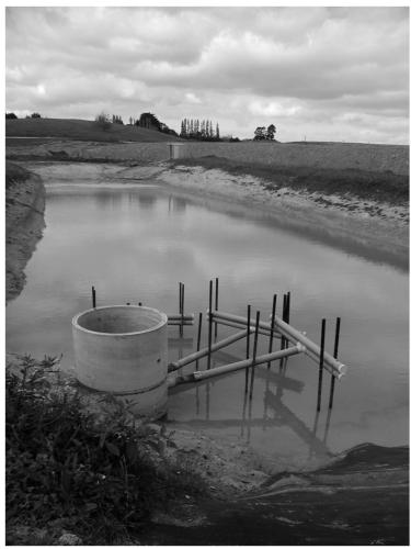
Figure 6-68. Multi-level, perforated, floating discharges (decants) to better retain floc.
