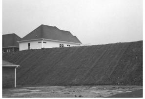
Slope being protected with netting after failure
