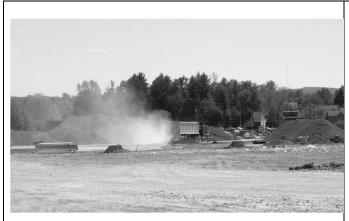
In this commercial mall rehabilitation project, dust became a problem even though much of the site area was impervious. Complaints were received from homeowners beyond the work area in the direction of the prevailing winds.
