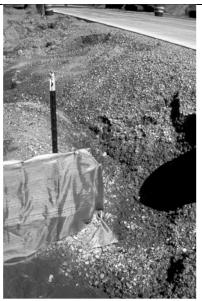
Flows commonly erode around ends of filter fabric check dams
