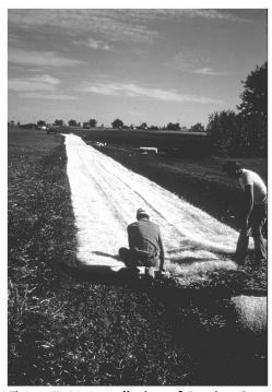
Figure 5-44. Installation of Erosion Control Matting (SCS photo)
