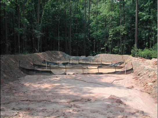
Figure 6-3. Dry pond at construction site with baffles (Source: McCaleb, et al. 2008).
