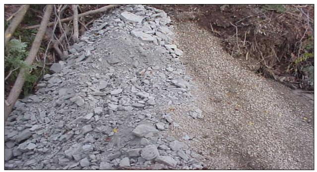
Figure 6-76. This is a stone check dam faced with pea gravel to slow water velocity and trap sediment (D. Lake photo)
