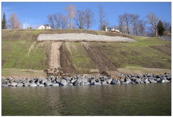
Figure 5-66. Additional stabilization methods included the use of willow live stakes as a biotechnical slope stabilization measure (T. Cassel photo)
