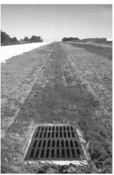
Figure 4-25. Sodding, or other reinforcement, is usually needed along concentrated flow pathways
