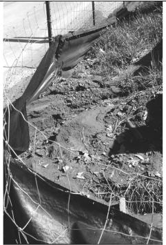
Inspections must enforce needed maintenance before failure. This silt fence is retaining massive amounts of sediment and is near its limit and needs to be maintained soon.
