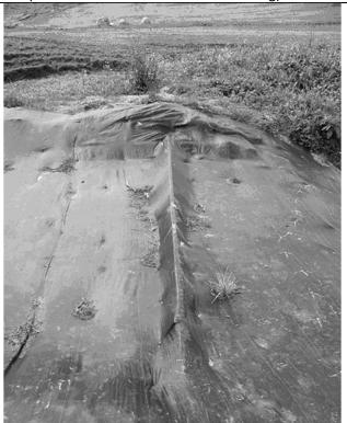
Temporary outlet made from timber placed at correct elevation and covered with plastic trap to protect spillway (Auckland Regional Council)
