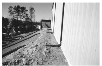
Figure 2-18. Small-scale slope diversion to safely carry roof runoff away from building and down sensitive adjacent slope.
