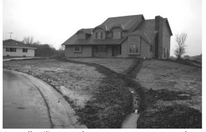
A small utility trench can cause concentrated flow resulting in greater erosion
