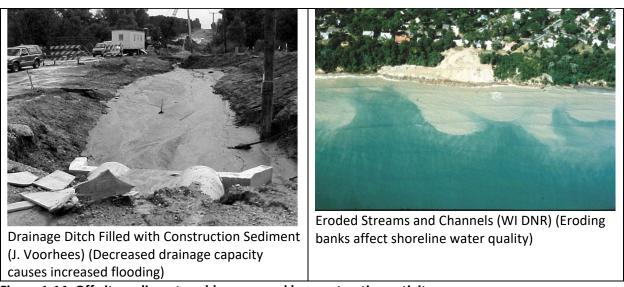
Figure 1-14. Off-site sediment problems caused by construction activity.
