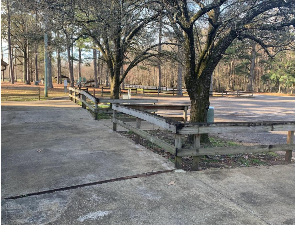
Figure 1.2 Cracked concrete sidewalk damaged from root growth elevating the slab 2 inches and causing trip hazards for pedestrian traffic
