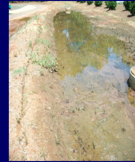
Extended ponding of water in low area of biofilter after rain.
