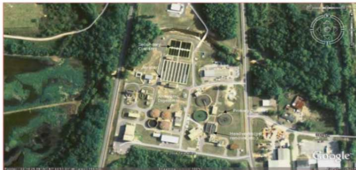
Figure 1. Hilliard K. Fletcher Wastewater Treatment Plant
