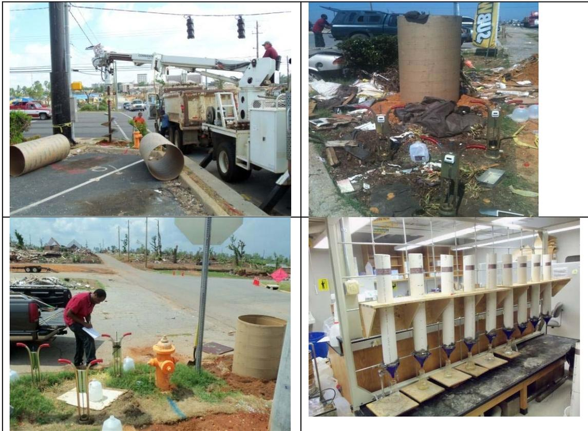
Figure 4. Photographs showing borehole drilling, Sonotube infiltration tube installation, double-ring infiltration measurements, and laboratory column tests.
