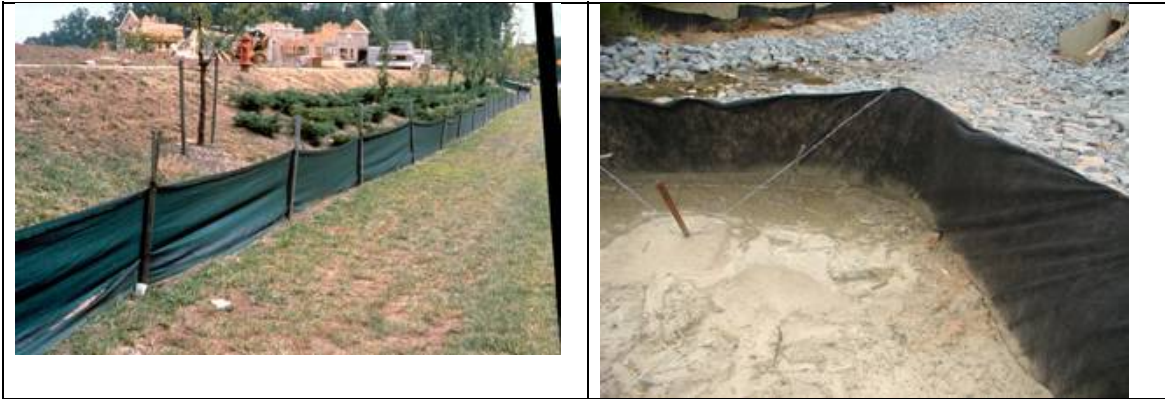
Filter fencing for small drainage areas
