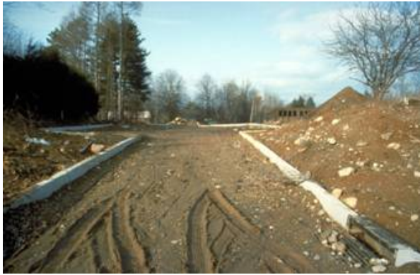
Control of runoff is critical at the beginning of construction. Here the stormwater infrastructure is in place but the 24 inch storm sewer is 75% plugged with sediment. Note the size of the material on the catch basin grate.
