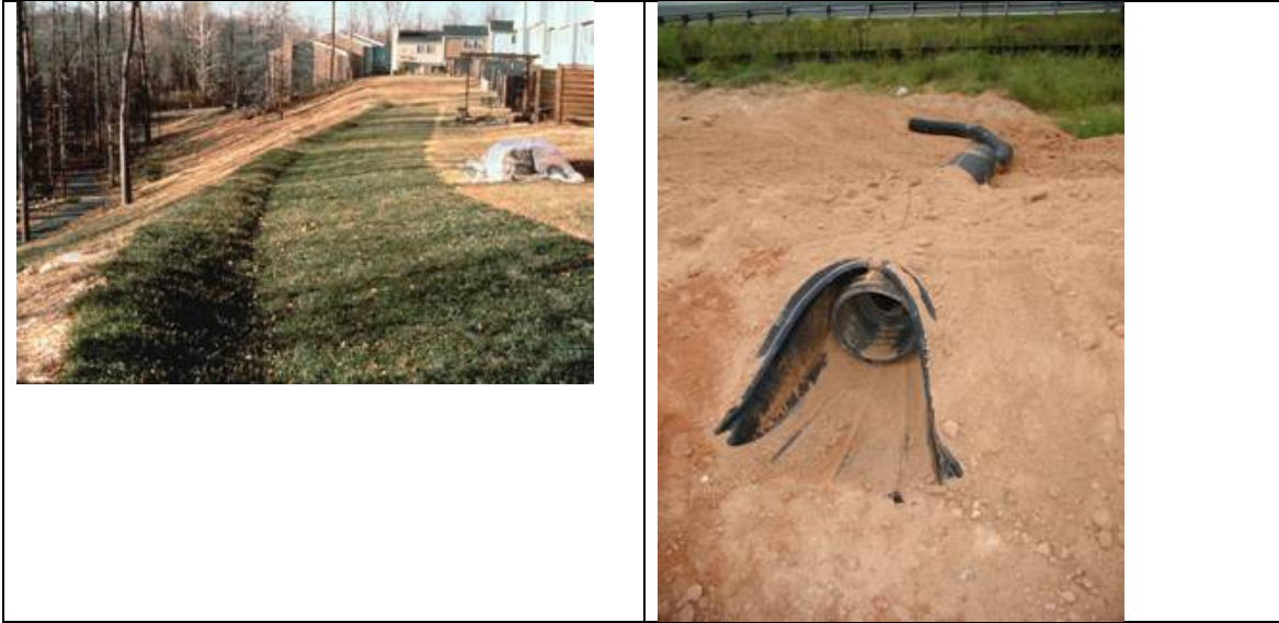
Diversion of Flows
