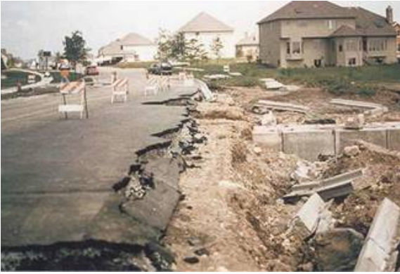
Damage from Erosion Requiring Repairs (IECA photo)
