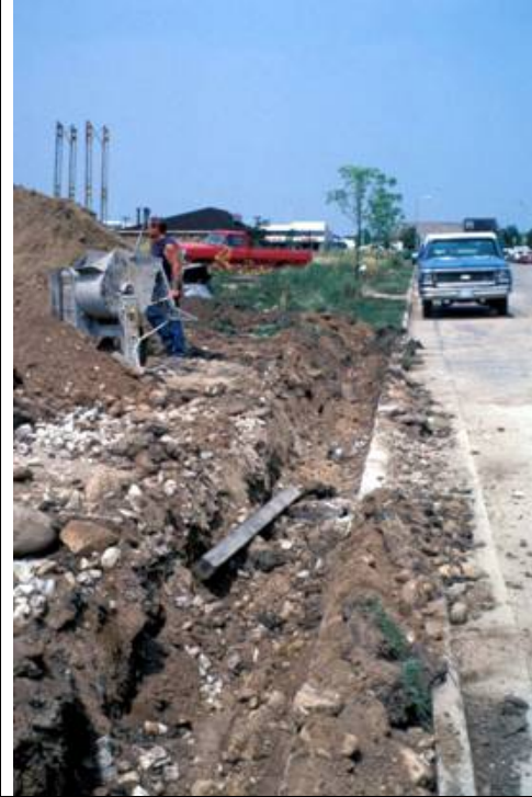
Stock Pile Problems and Working Close to Roads
