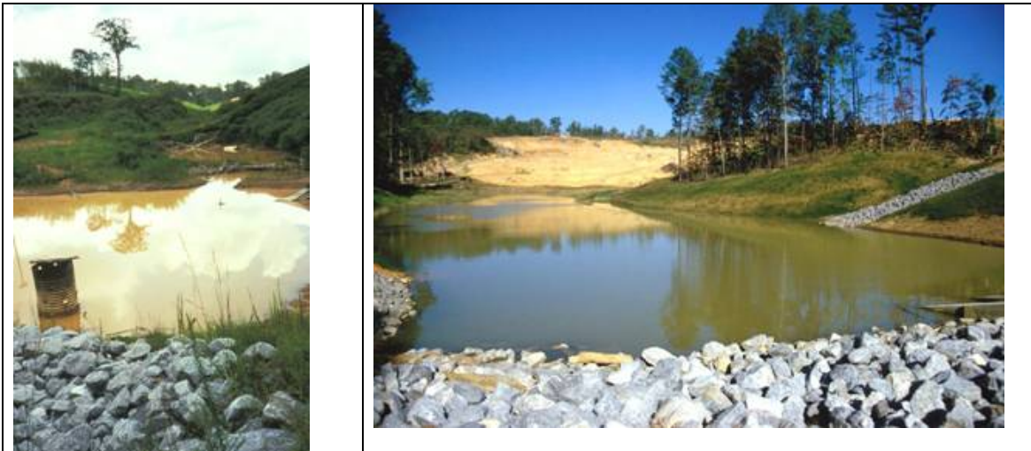
Sediment ponds for larger areas
