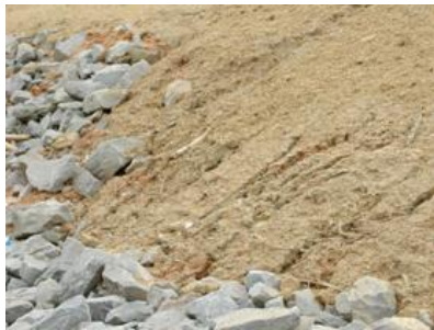
Failing Mulch on Slope above Rip Rap
