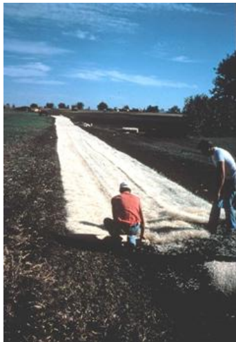
Installation of Erosion Control Matting (SCS photo)
