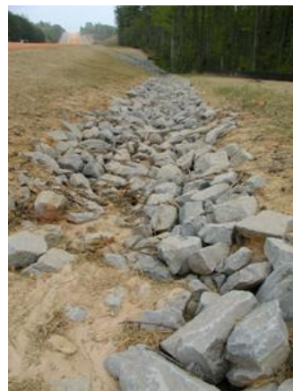
Close-up of rock reinforced channel, showing sediment accumulation between rocks.
