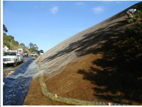
Installation of Wire Netting over Mulch
