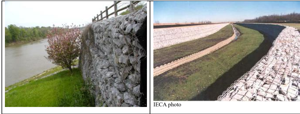
Gabion Wall Channel Protection
