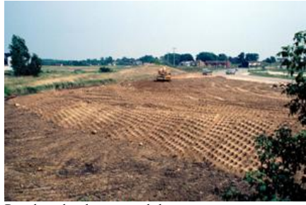
Roughened and compacted slope. Soil Roughening to Protect Slope
