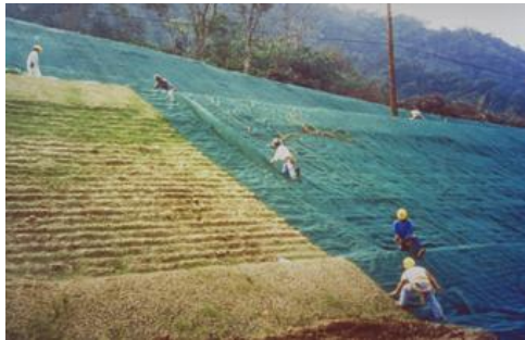
Installation of Netting over Mulch
