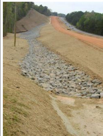
Large rocks for channel reinforcement
