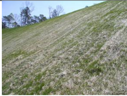
Slopes Protected by Erosion Control Netting and Vegetation
