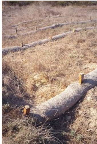
Coir rolls/logs and soil adhesives for slope stabilization project at Newport Beach, CA, wildlife refuge.
