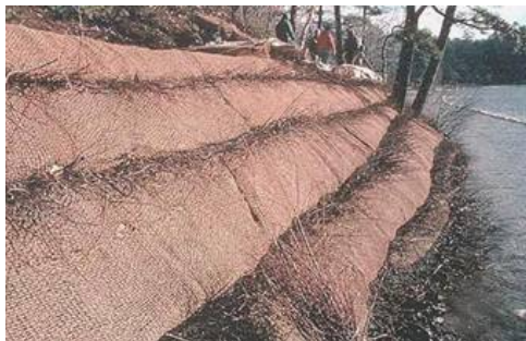
Bioengineered channel slopes (IECA photo)
