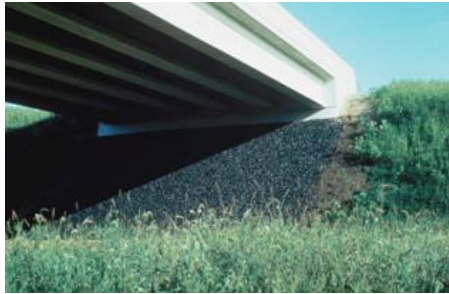
Asphaltic Slope Protection in Heavy Shade
