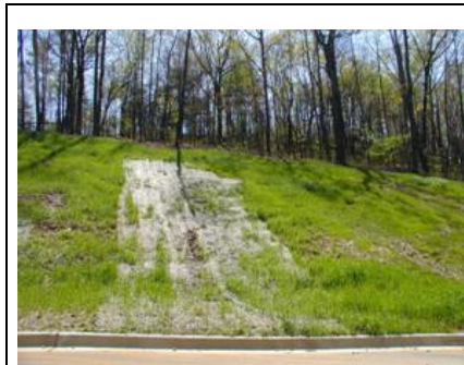
Failing Mulch on Slope above Rip Rap
