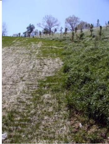
Reinforced slope netting and established vegetation at Birmingham, AL, highway project.
