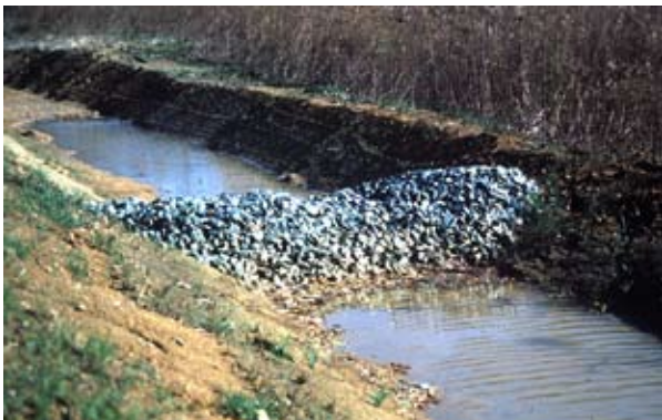
Examples of rock check dams
