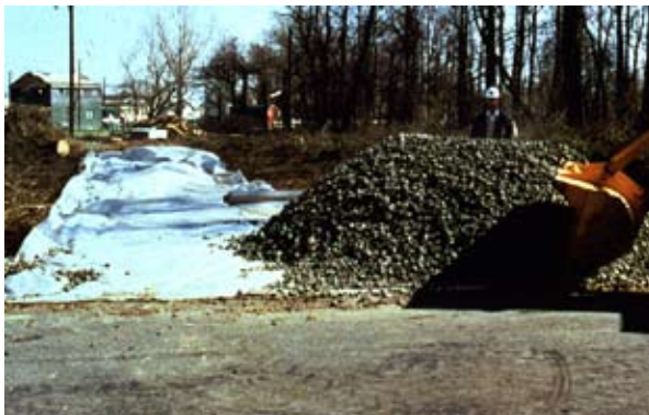
Stabilized construction entrance
