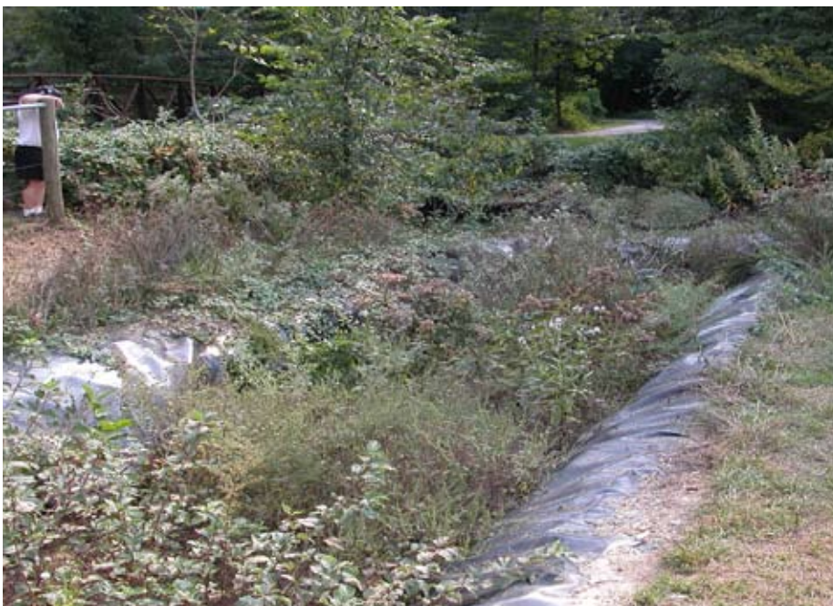
University of Maryland rain garden monitoring site
