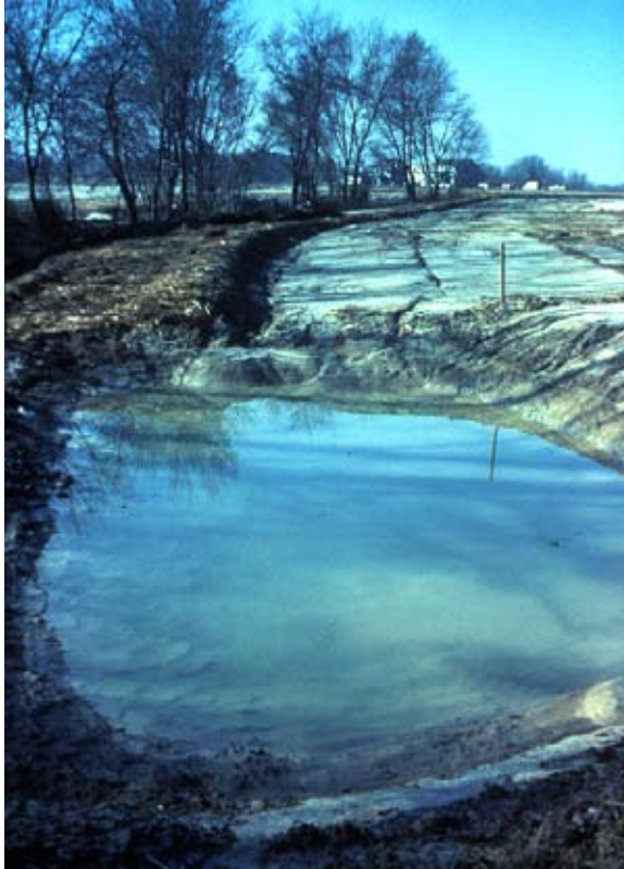
Sediment ponds and traps
