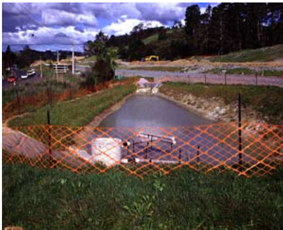
Sediment ponds and traps
