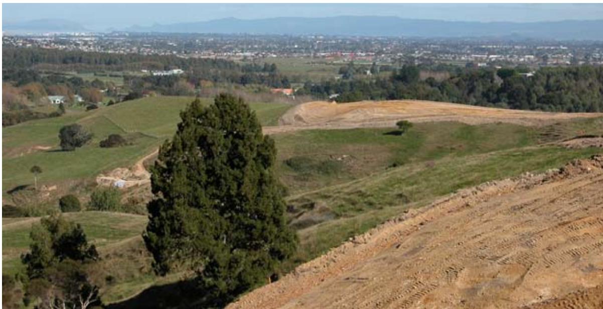
Minimal disturbance for earthmoving
