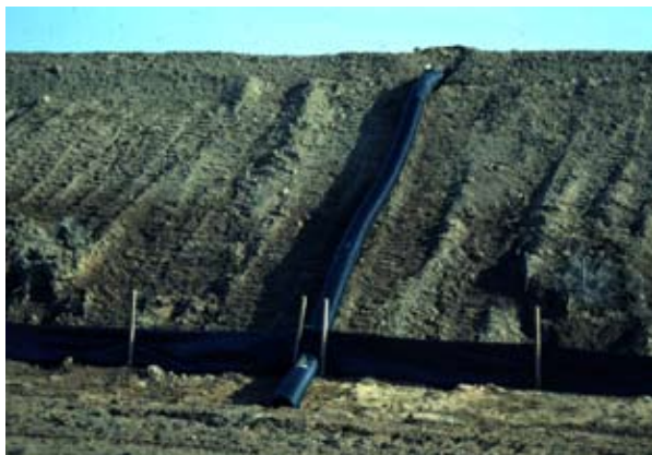
Examples of pipe and flume downdrains
