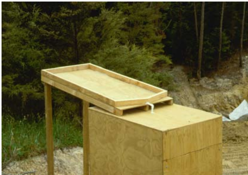
Roof area of flocculation unit
