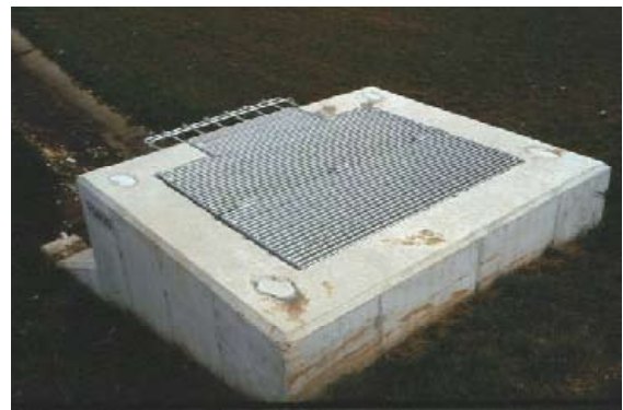
GOOD: Lightweight, noncorroding aluminum top gratings are safe to stand on and easy to lift.
