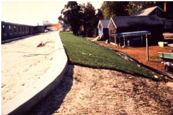
Turf being applied to topsoil
