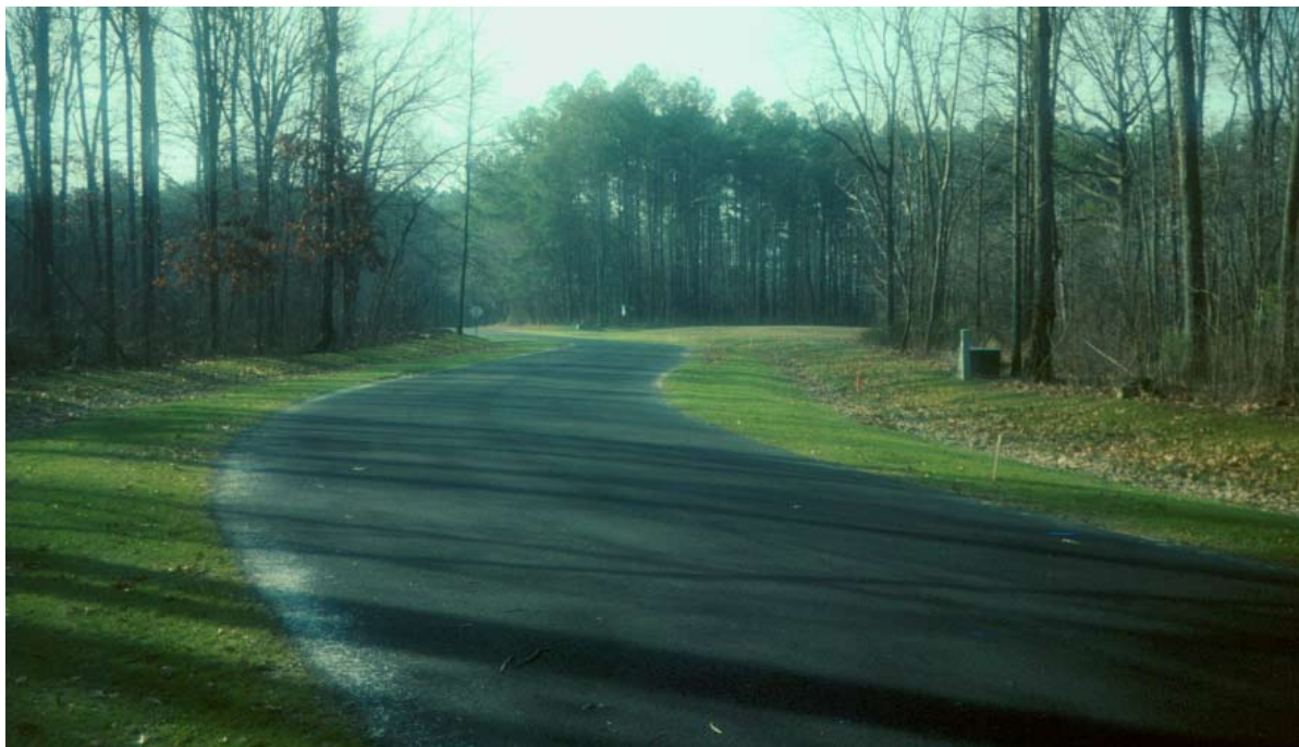
Subdivision without curbing or catch pits
