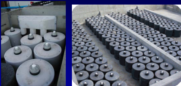
Contech Solutions Storm Filter, the most commonly used stormwater filter in the US, is used to treat runoff from roof drains to airports.
