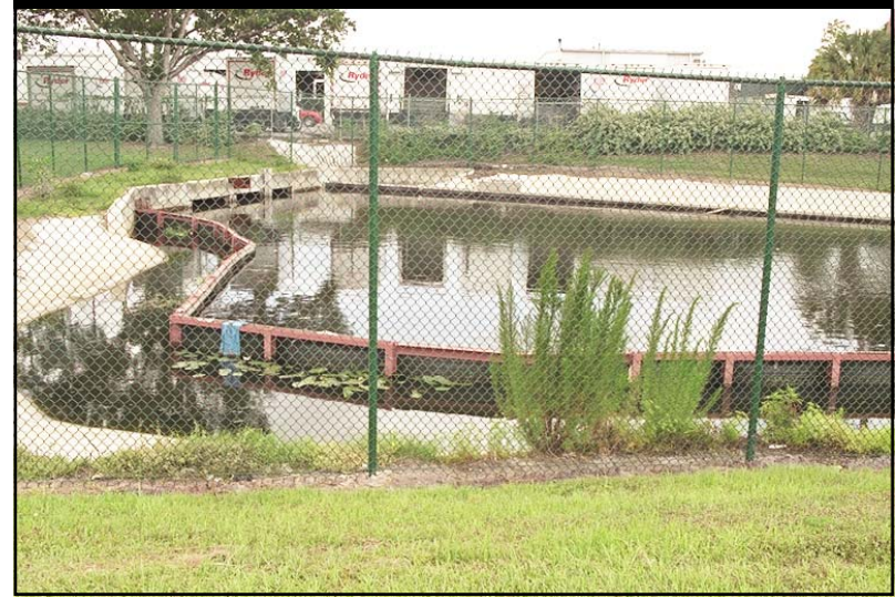
Settling Pond after Alum Injection, Orlando, FL
