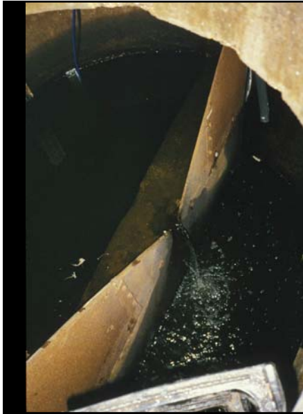
Modification of Outlet for Improved Performance
