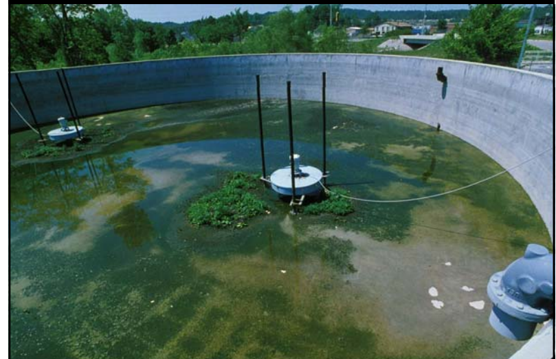
Equalizing Dry Pond to Control SSO Problems, Moody, AL
