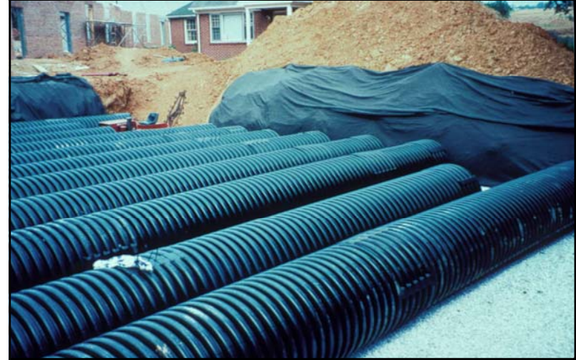
Large Corrugated Pipes used for Underground Detention Below Parking Area
