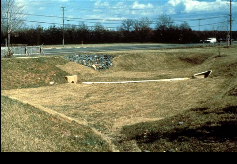
Typical Dry Detention Pond, with Pilot Channel
