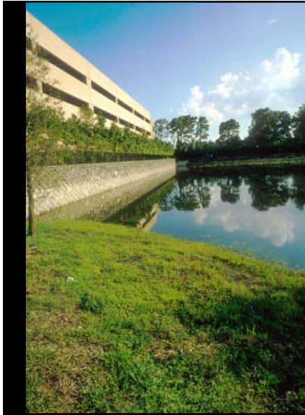
Wet Detention Facility at Convention Center, Orlando, FL
