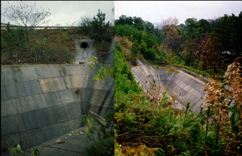
Unusual Dry Detention Pond Located on Hillside to Meet Peak Flow Rate Criterion
