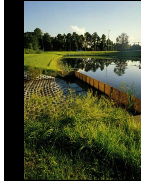
Modification of Pond Outlet at Epcot Center, Orlando, FL
