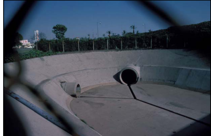
Dry Detention Pond Forebay for Stormwater Pump Station, Los Angeles, CA
