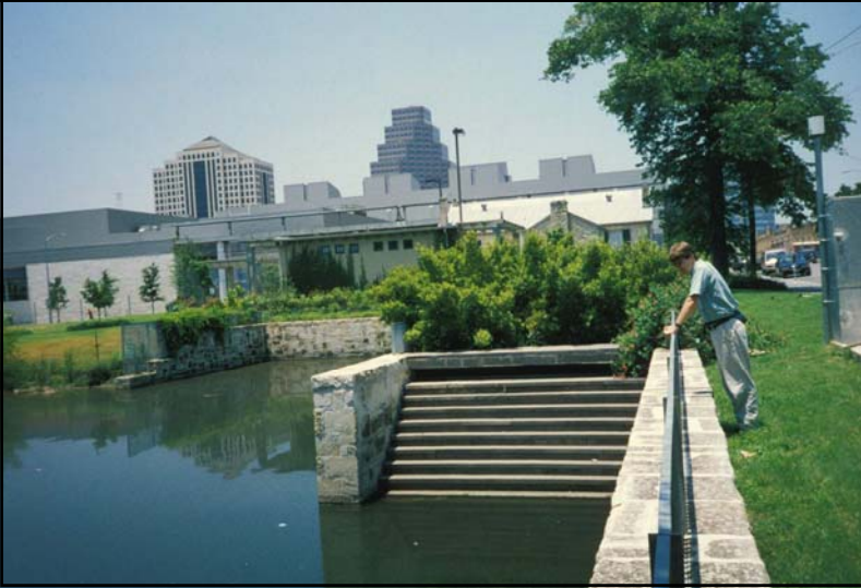
Wet Pond after Oil and Grease Trap and Step Aerator, Austin, TX
