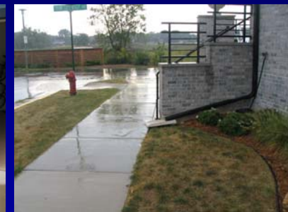
Directly connected roof drain
