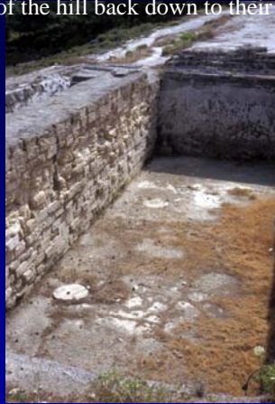
Cistern tank, Kamiros, Rhodes, collected roof runoff from adjacent temple located at top of the hill.
