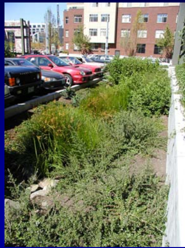
Parking lot biofilter example, Portland, OR
