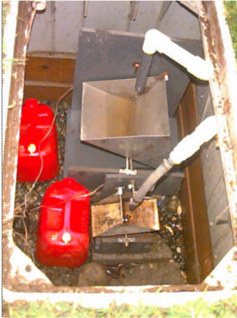
Figure 2-5. Picture of the tipping bucket installation for monitoring surface runoff and subsurface flows at the University of Washington
