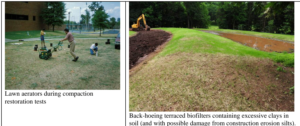
Figure 6. Less successful mechanical soil restoration efforts.
