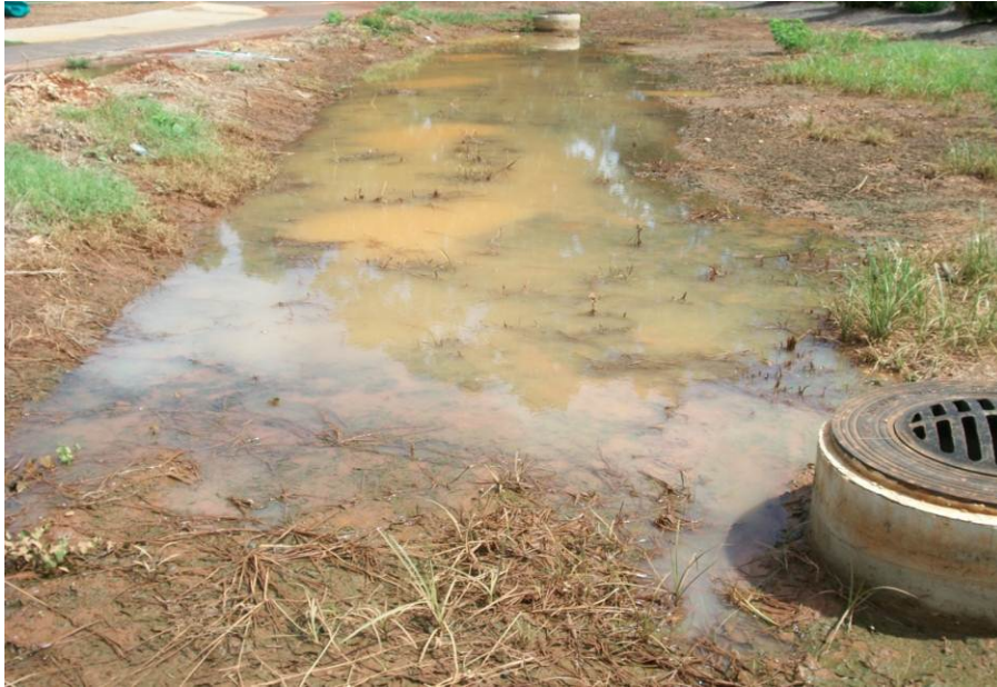
Figure 7. Ponded water on the biofilter surface observed after rainfall event (the vegetation cover is very poor indicating likely serious compaction).
