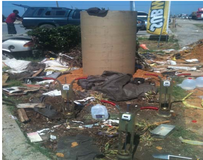
Figure 2. Double Ring Installation at Test Site 1.
