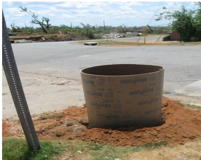
Figure 5. Borehole Installation at Test Site 3.
