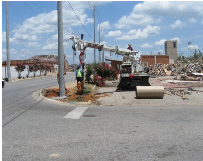
Figure 4. View of Borehole Drilling at Test Site 3.
