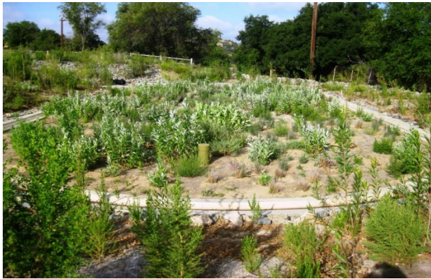
Figure 5. Lower Parking Lot Sedimentation Basin and Biofilter
