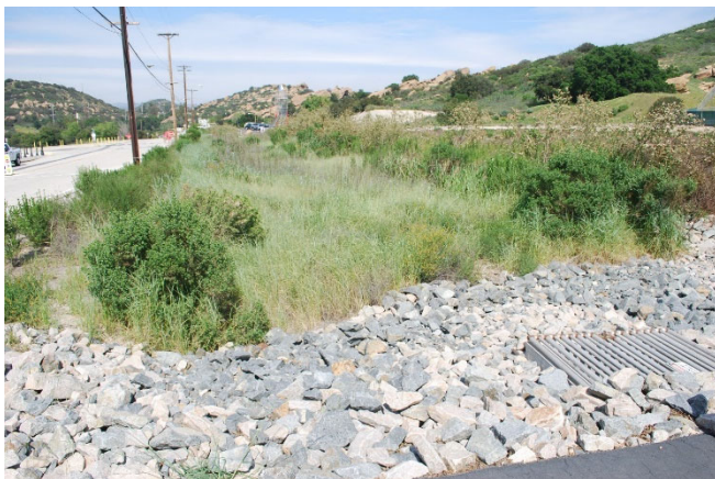
Figure 4. B1436 Detention Bioswales
