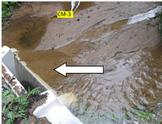
Figure 35. Sediment accumulated behind weir boards at CM-3.
