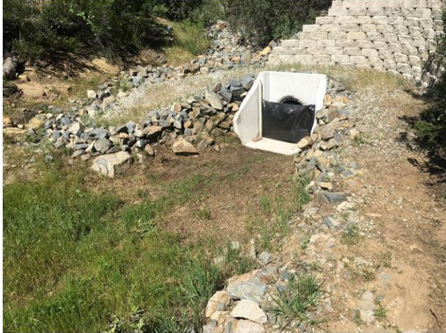
Figure 16. Culvert modifications installed in 2009.
