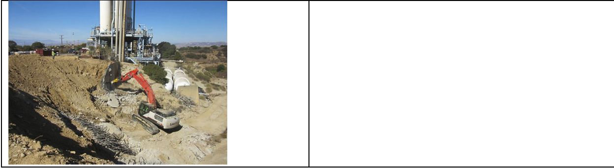
Figure 2. Photos of Phase 4 demolition from NASA website (NASA b)
