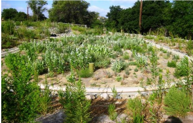
Figure 18. Lower parking lot sedimentation basin and biofilter installed in 2013.
