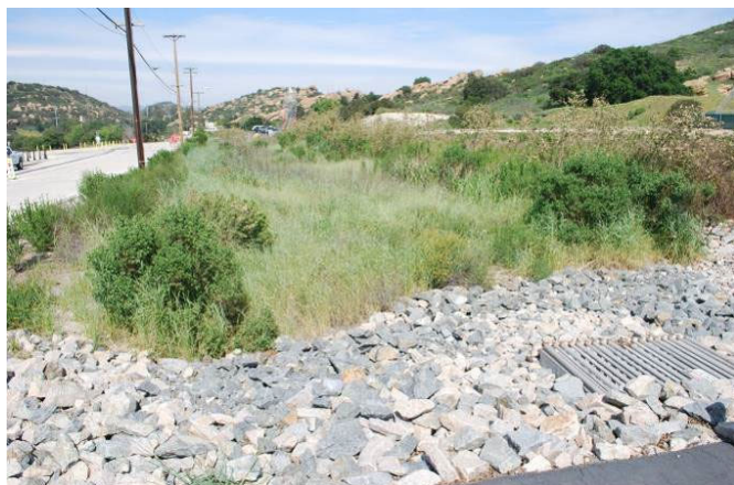
Figure 20. Detention bioswales installed in 2015.
