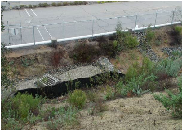
Figure 17. B-1 Sedimentation basin and media filter installed in 2012.
