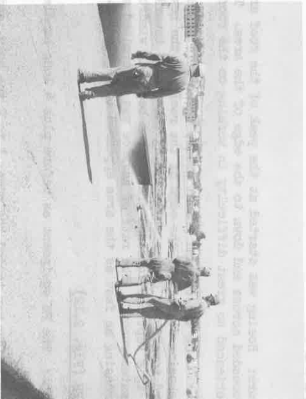
FIG. 2.11 Firehosing and Hand Scrubbing Roof Area.
