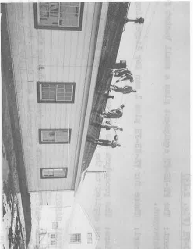
FIG. 2.11 Firehosing and Hand Scrubbing Roof Area.
