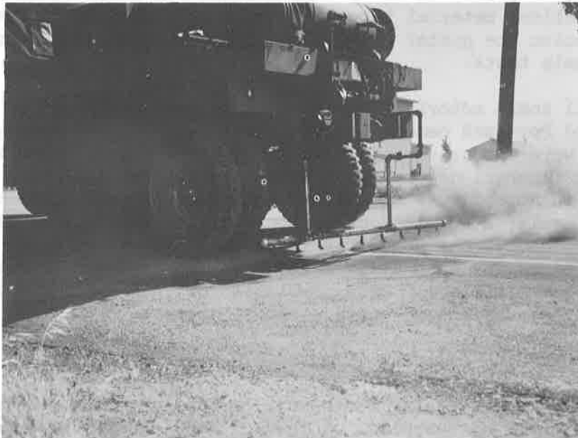
Fig. 2.3 Vacuumized Sweeping (Tennant Model 80) on Asphaltic Concrete.
