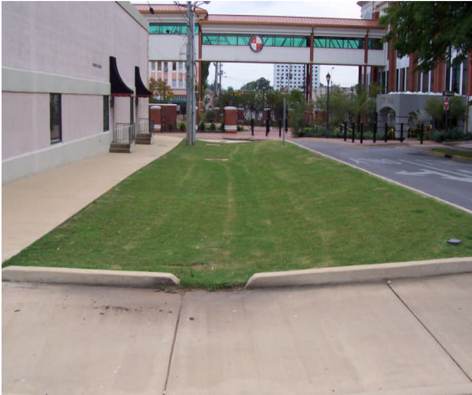
Figure 79. Picture showing the outdoor test swale (116 ft (35.3 m) in length draining 0.1 acres (390 m 2 ) of paved road).
