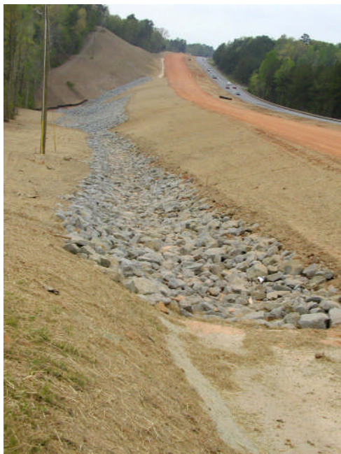
Large rocks for channel reinforcement and to reduce the velocity.
