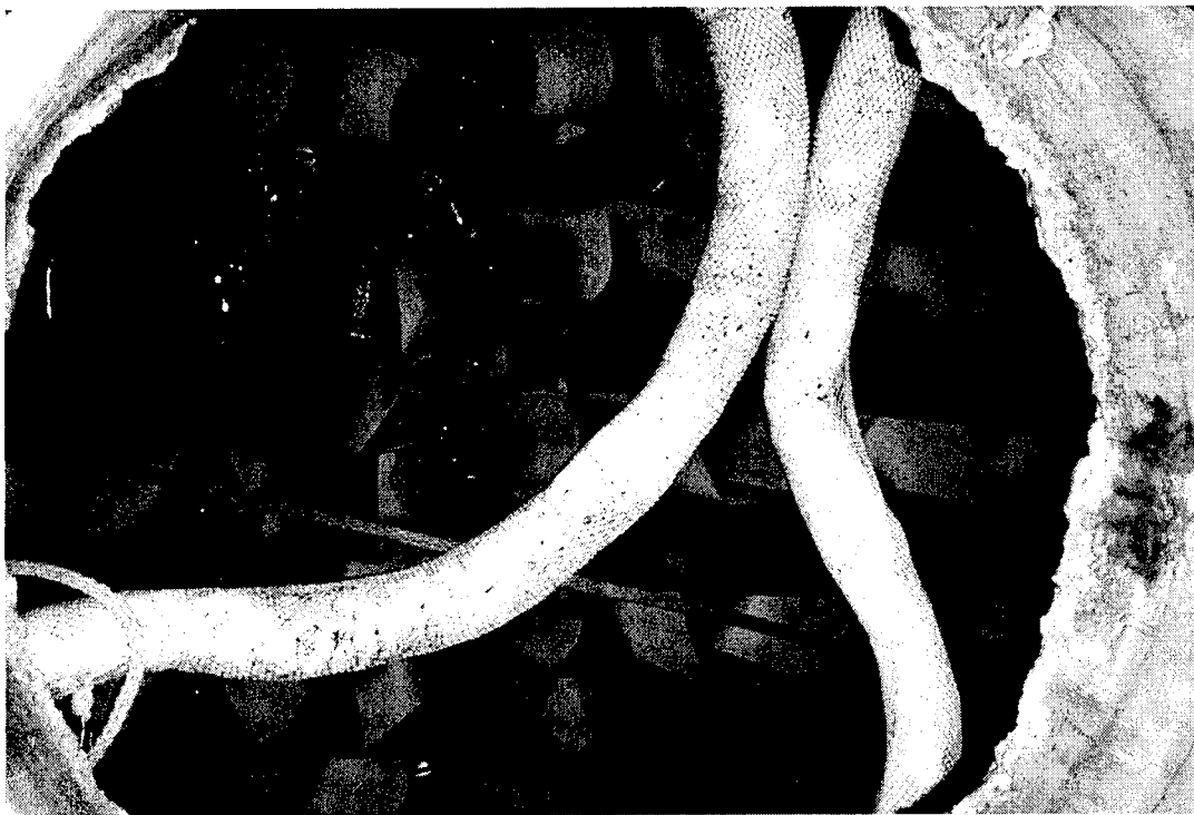
Figure 5.14 Ruby Garage, Milwaukee, MCTT main settling chamber inclined tube settlers and sorbent pillows (WI DNR photo).
