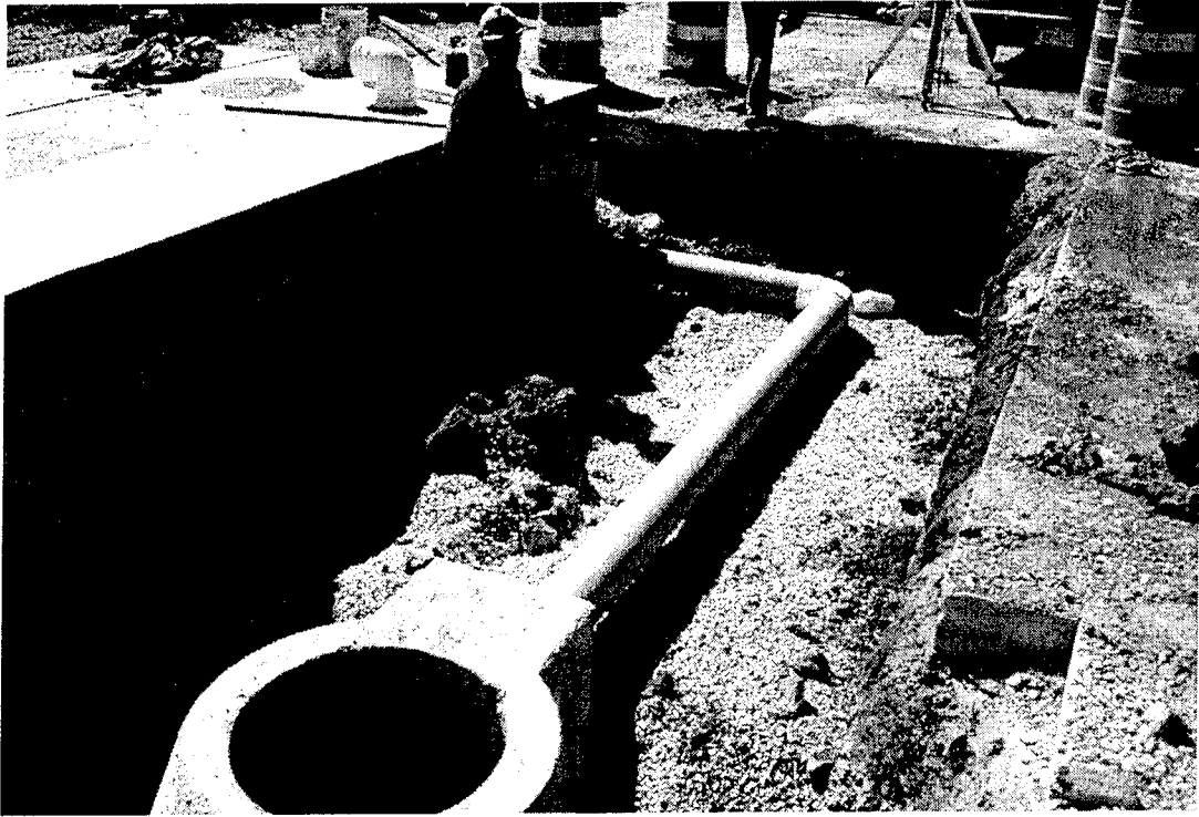
Figure 5.13 Ruby Garage, Milwaukee, MCTT catchbasin inlet and piping (WI DNR photo).
