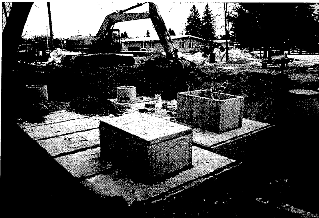
Figure 5.17 Minocqua, WI, MCTT, installation of box culverts (WI DNR photo).
