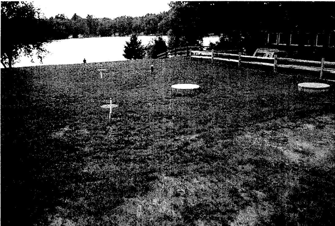
Figure 5.22 Minocqua, WI, MCTT, site after installation.
