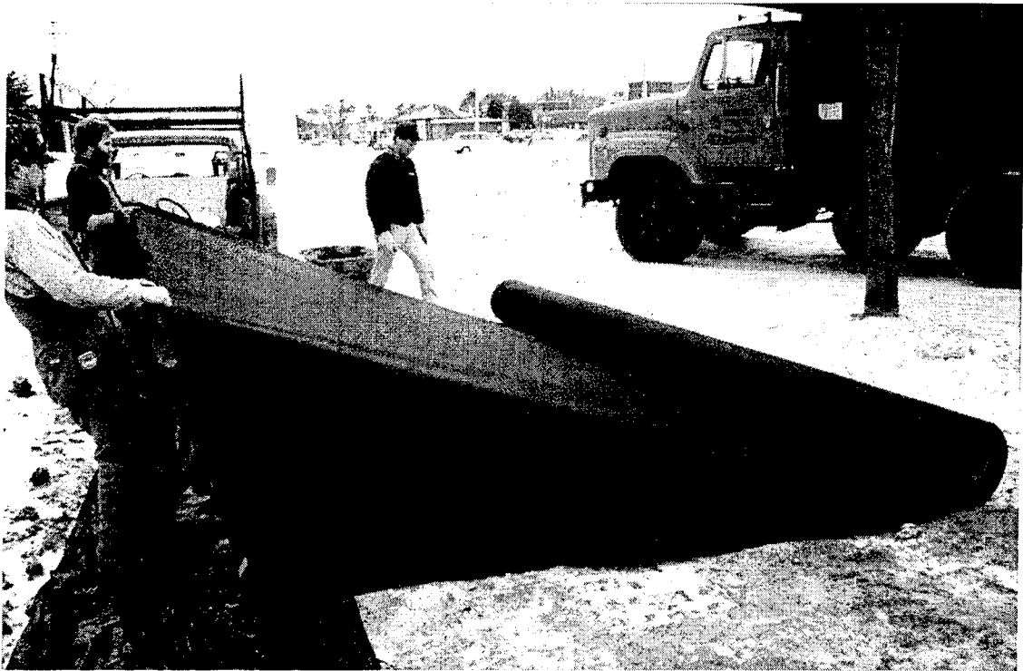
Figure 5.19 Minocqua, WI, MCTT, filter fabric being prepared for installation (WI DNR photo).
