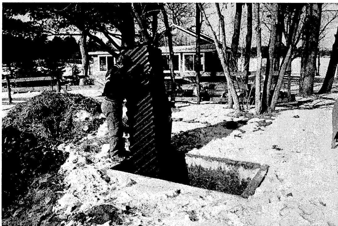
Figure 5.18 Minocqua, WI, MCTT, placement of tube settlers (WI DNR photo).
