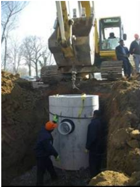
Figure 3. Installation of Tuscaloosa UpFlo™ filter.
