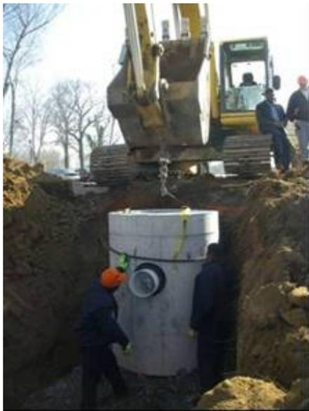
**Figure 3. Installation of Tuscaloosa Up-Flo<sup>®</sup> filter.**
