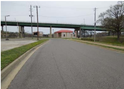
Only one building at the site with small roof area
