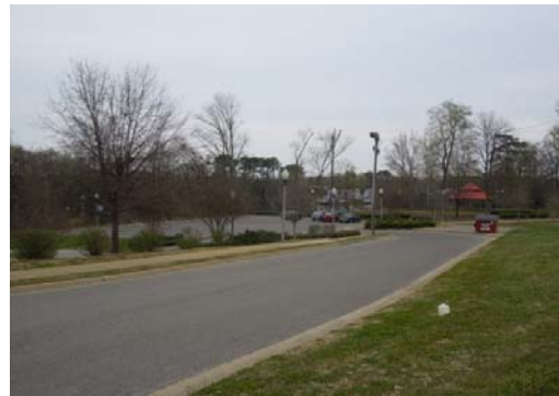
Slight slope along the parking lot entrance road directs the runoff into the parking area and filter
