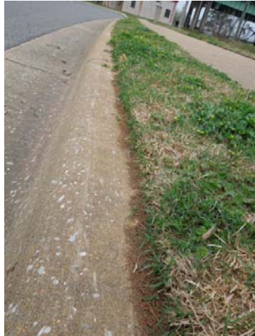
Eroding soils beside the roadway near the filter inlet due to fire ant activity
