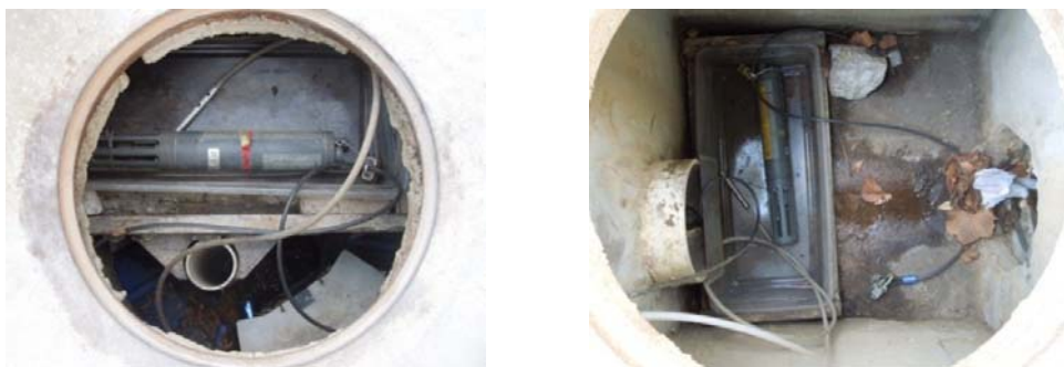
Figure 5: Pre-Storm Field Setup and Cleaned Plastic Trays of Influent and Effluent
