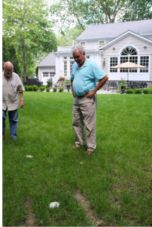
Backyard dry well at new home on Tennyson Rd. used for water quality monitoring (monitoring well caps shown), sealed against surface inflows.
