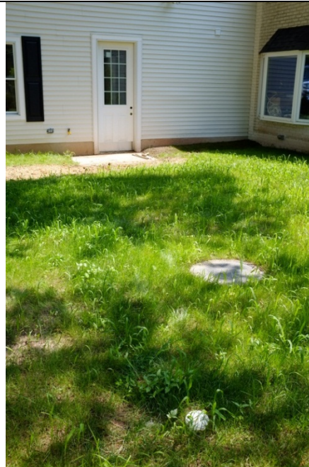
Backyard dry well at new home on Parsonage Hill Rd used for water quality monitoring; sealed against surface inflows.
