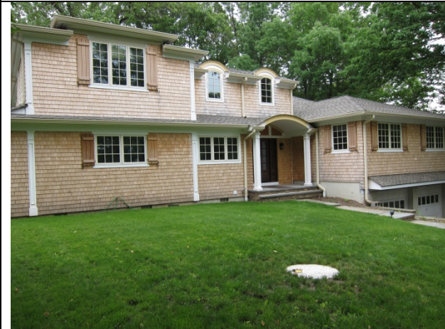
Front yard dry well only receiving roof runoff.
