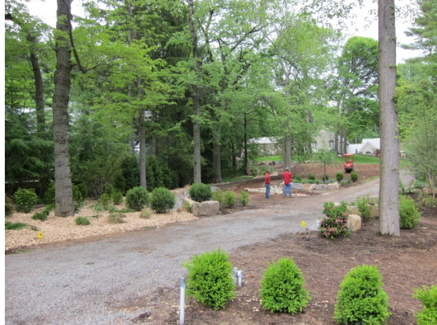
Landscaping in yard having underground cistern.
