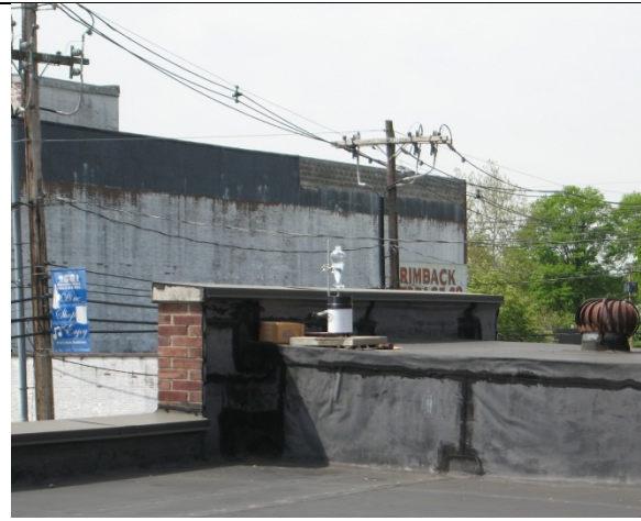
R2: Roof of Township's maintenance garage (gage being calibrated)
