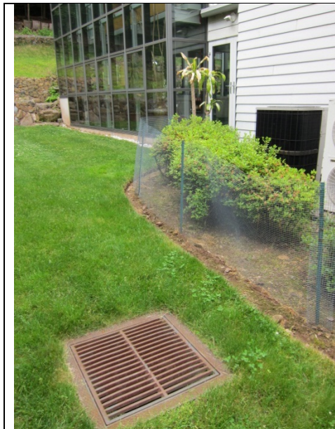
Backyard dry well showing lawn area also as a source.
