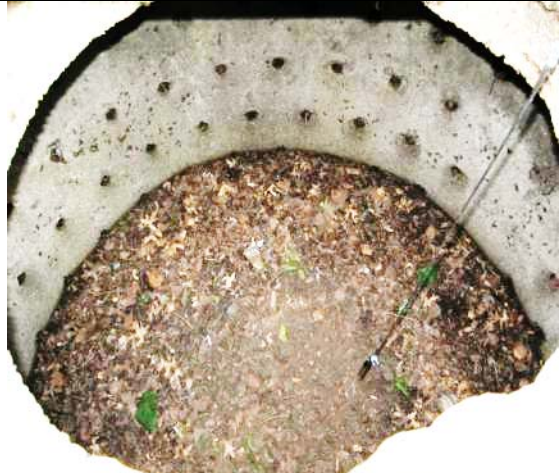
Dry well (258 Main St.)
