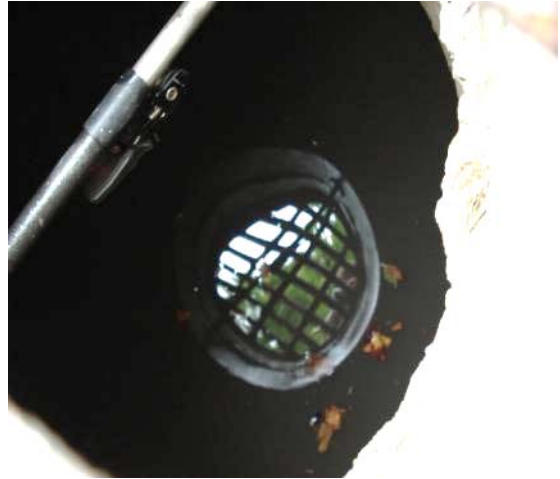
Dry well with standing water (383 Wyoming)
