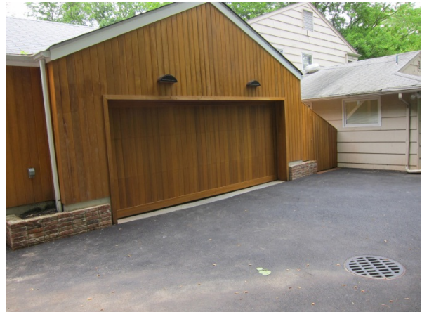
Backyard dry well on Wyoming St. showing driveway runoff also as a source.
