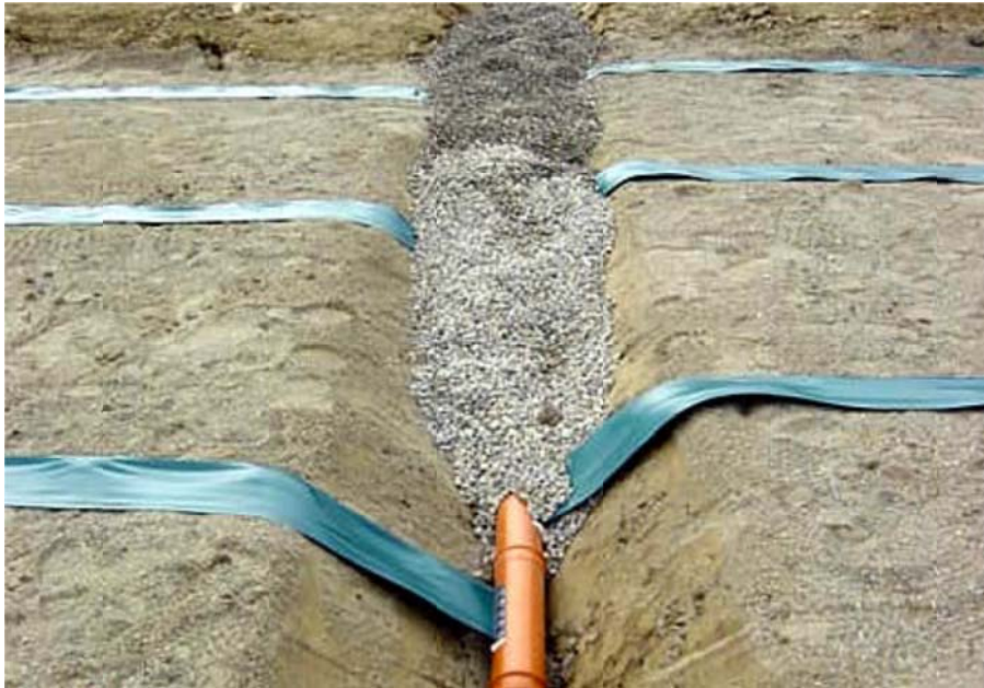
Figure 15. The SmartDrain Belt® System during Construction (Morhard 2006).
