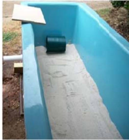
(b) SmartDrain™ showing underlayer of sand
