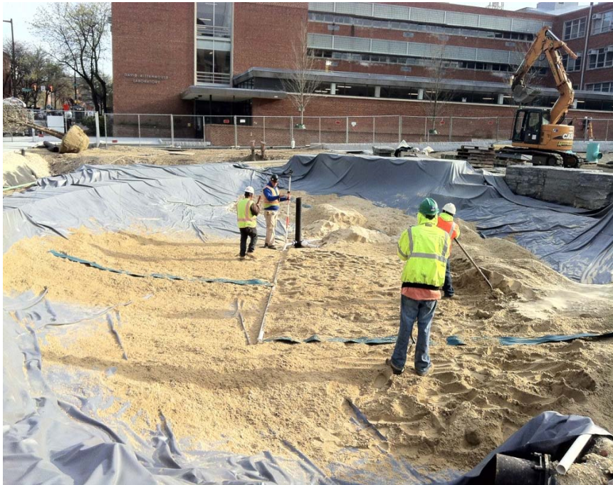
Figure 12. SmartDrain™ Installation at the University of Pennsylvania Shoemaker Plaza Project.
