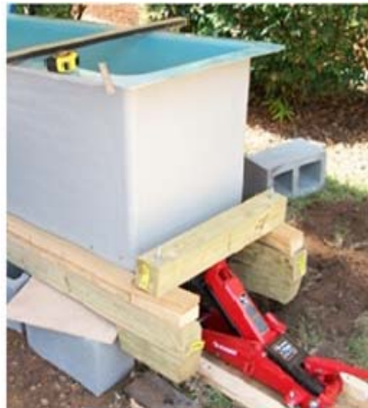
(d) A Hydraulic Jack and Blocks Used to Change the Slope of the Trough
