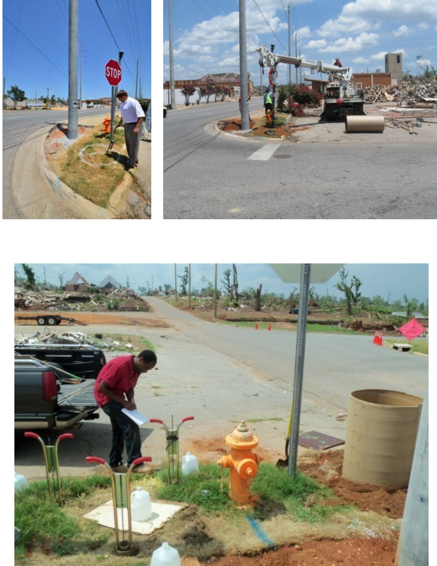
Figure 93. Borehole Marking, Borehole Drilling, and Borehole Infiltration Measurement Installations on 21 th Ave. and University Blvd E. (Alberta Hand Carwash).
