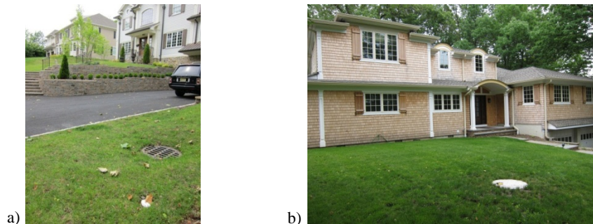
Figure 1.2 Typical Millburn dry well locations in front yards receiving lawn area inflows along with roof runoff.
