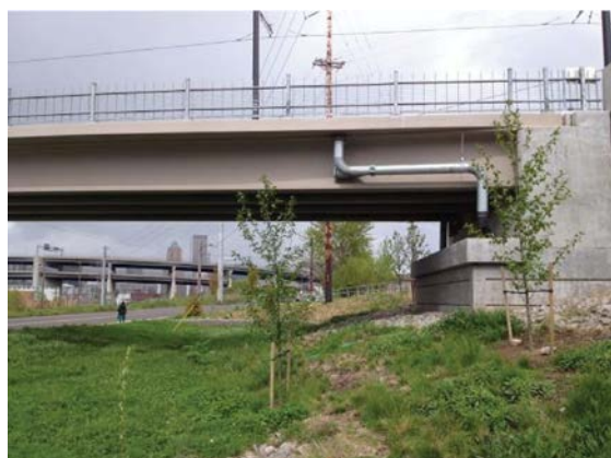
Highway 99E Viaduct, Portland, Oregon. (Photo credit: Geosyntec Consultants.)
