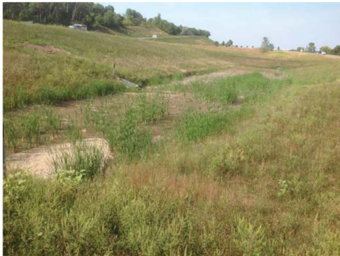
Figure 19. Sedimentation in floor of Pine Bend infiltration basin after construction.
