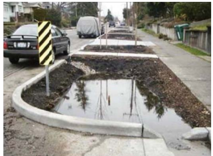
Figure 25. Examples of slowly draining rain gardens in the Ballard neighborhood of Seattle, Washington.
