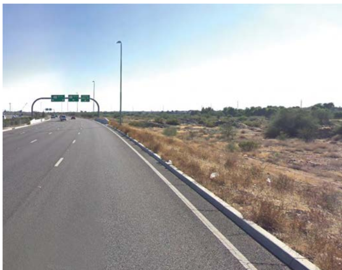
Figure 8. Example Phoenix, Arizona, freeway with sparsely vegetated shoulders.
