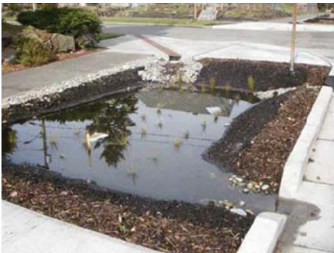
Figure 25. Examples of slowly draining rain gardens in the Ballard neighborhood of Seattle, Washington.
