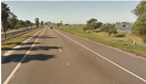
Informal dispersion to median and shoulder, Interstate 8, San Diego, California, urban area. (Credit: Google.)
