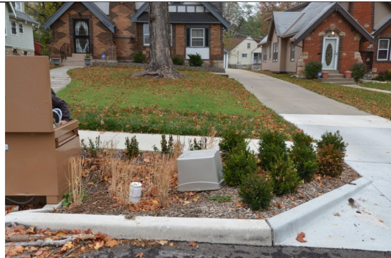
E edge of drainage area slopes away from rain garden (no house or driveway)
