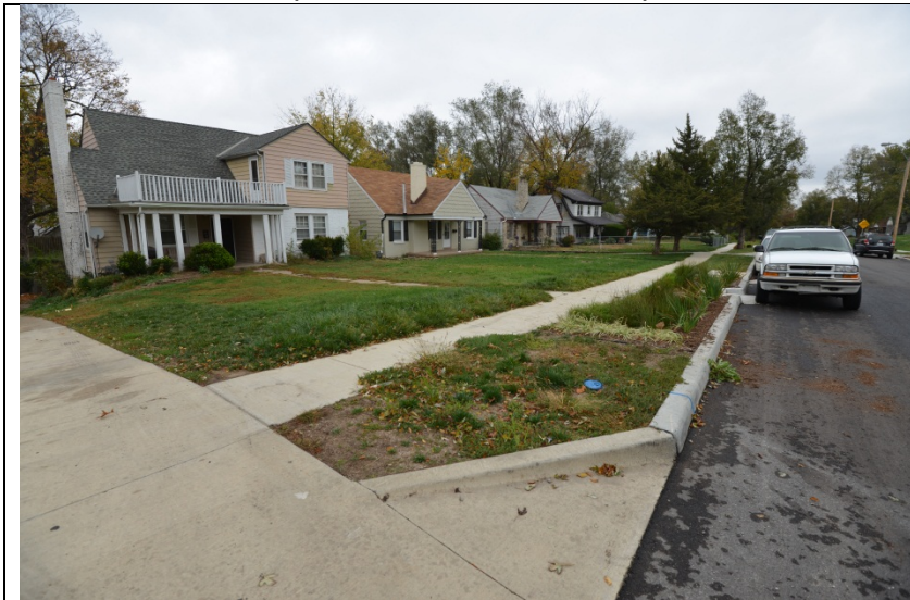
Towards E showing sloping driveway from rain garden; only half of street and a bit of yard to system (near top of street slope)
