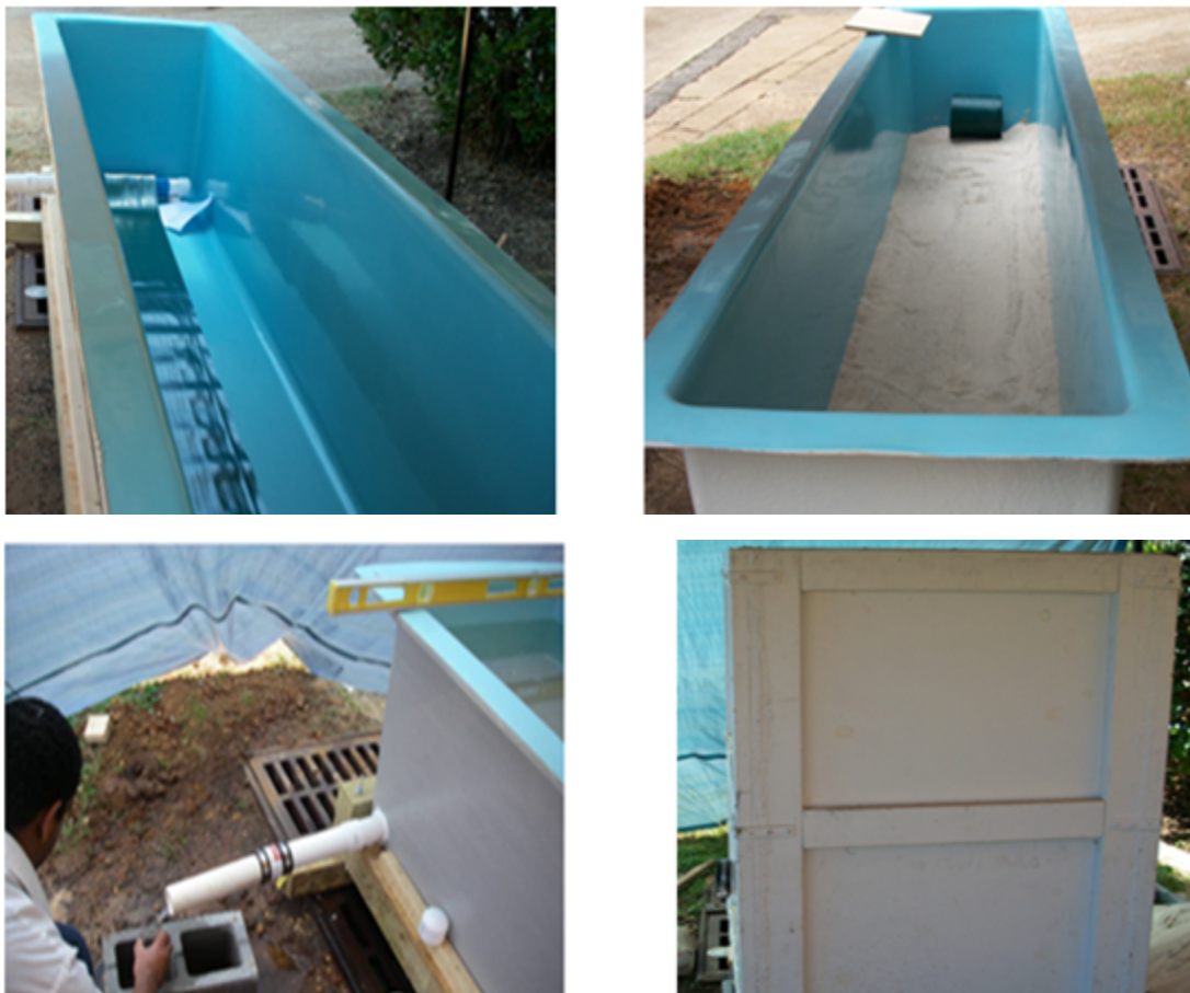
Figure 95. SmartDrain™ installation procedures in the trough.
