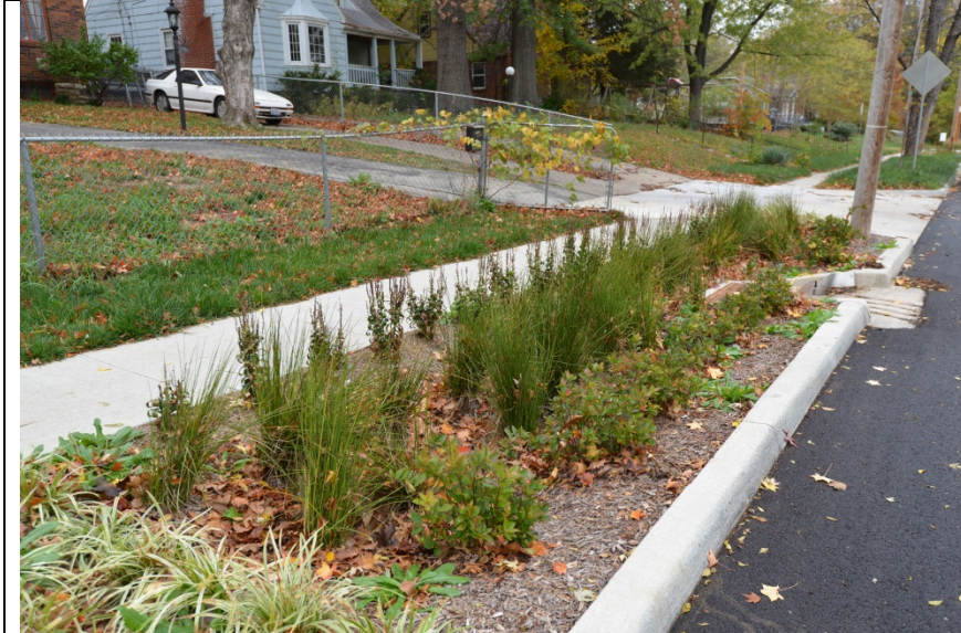
No samplers, 2 level recorders (inlet and bottom of rain garden)
