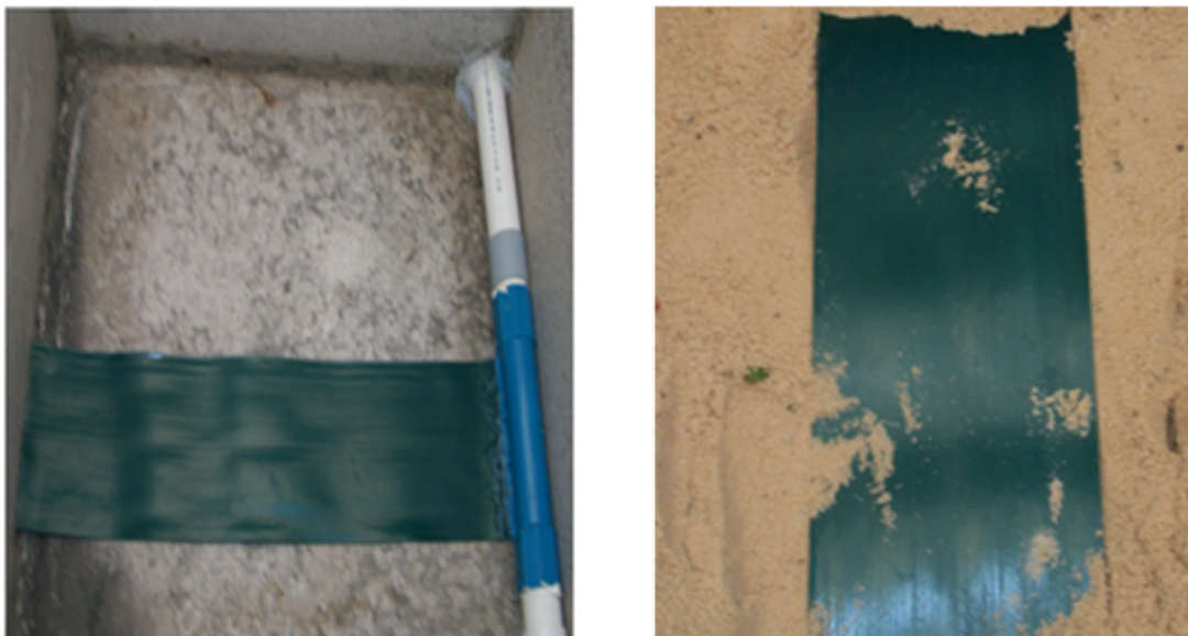
Figure 96. SmartDrain™ installation for the clogging test in the tall box.
