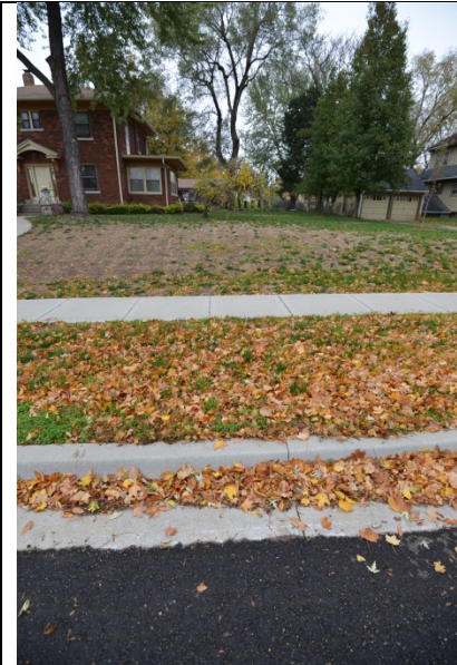
Drainage break to east (flows to left to device from edge of house)
