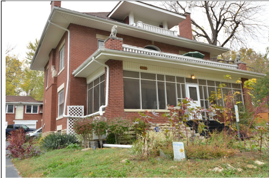
Roof drains from half of front and half of side of home
