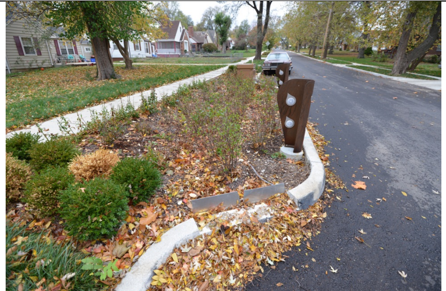
Looking upgradient towards Troost (most of lawns and homes slope south away from this location)
