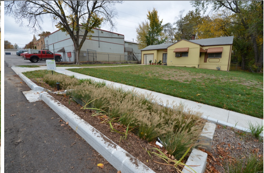
1112 E 76 th Terrace #9 (sheet 205 for as-built details); cascading swale (but upper weir set high so runoff bypasses other cells), no underdrains
