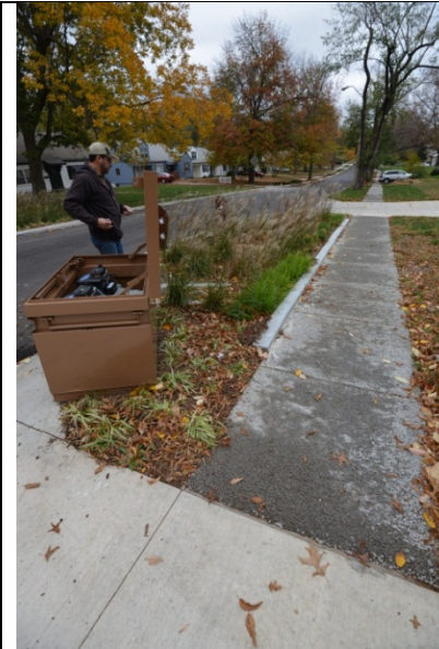
Porous concrete sidewalks all along street from Lydia to monitored rain garden
