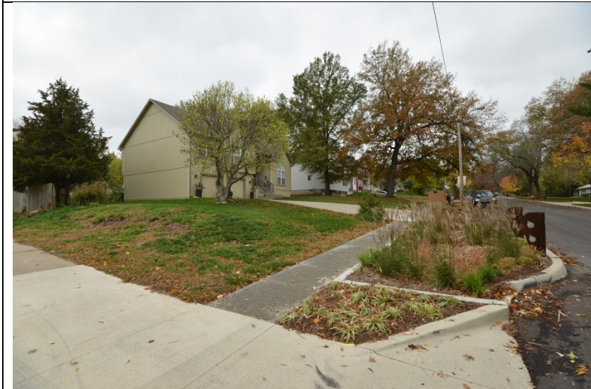
Showing bottom edge of drainage area
