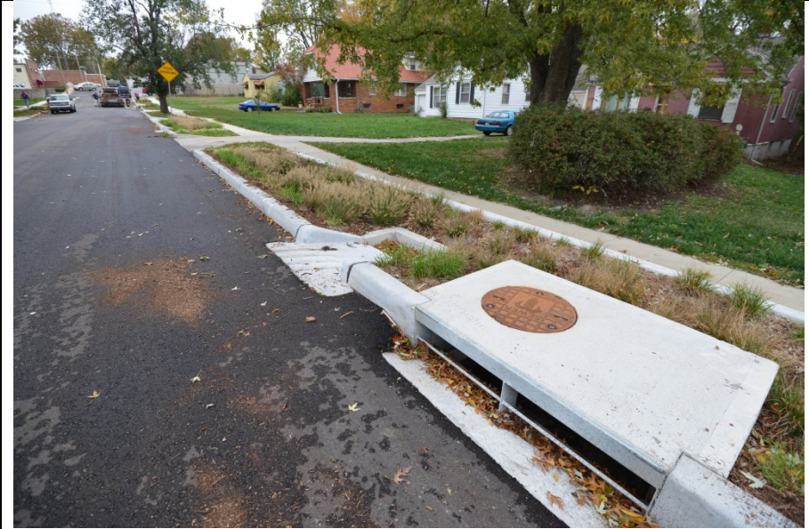
Very small drainage area; large inlet right below rain garden
