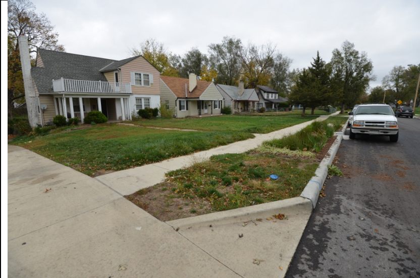
Towards E showing sloping driveway from rain garden; only half of street and a bit of yard to system (near top of street slope)
