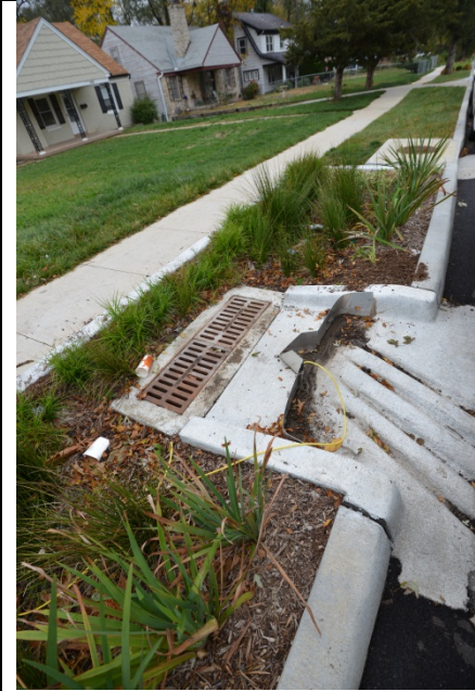
No samplers, but 2 level recorders at inlet and bottom of rain garden
