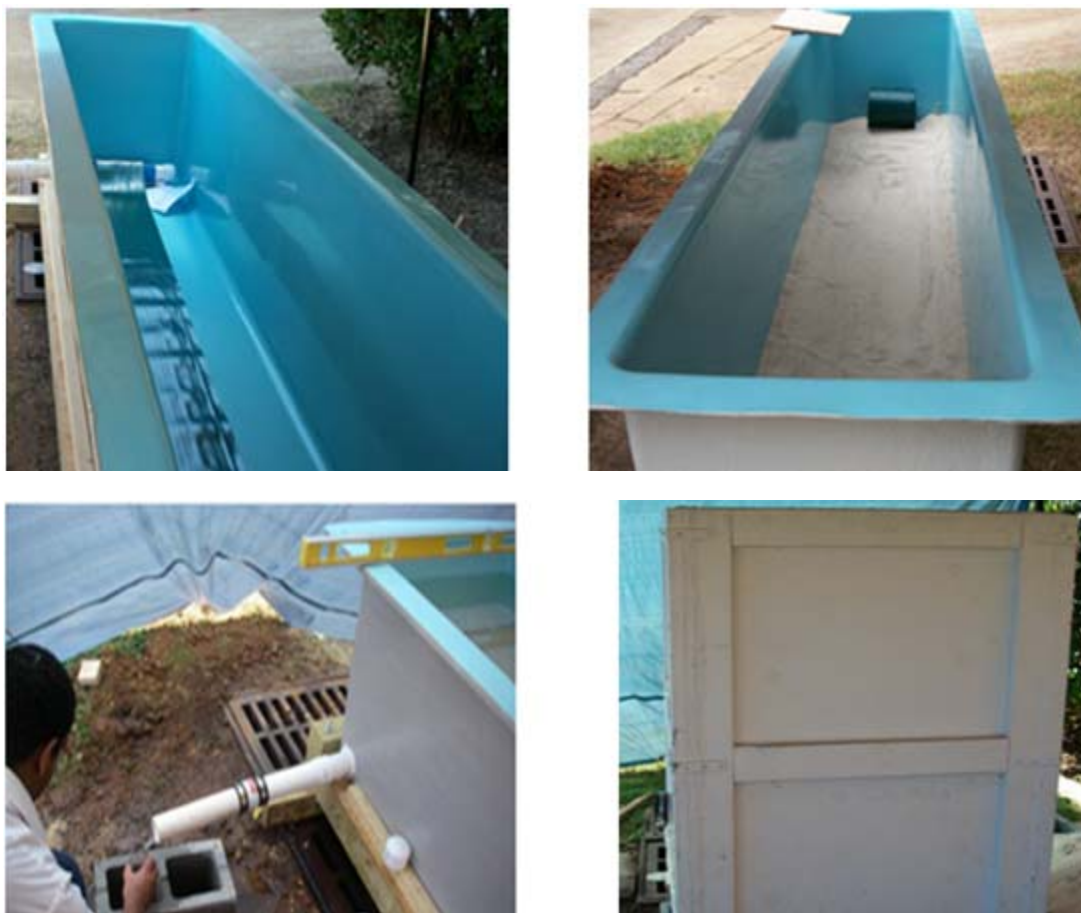
Figure 108. SmartDrain™ installation procedures in the trough.
