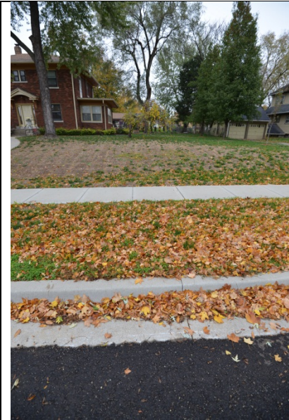
Drainage break to east (flows to left to device from edge of house)
