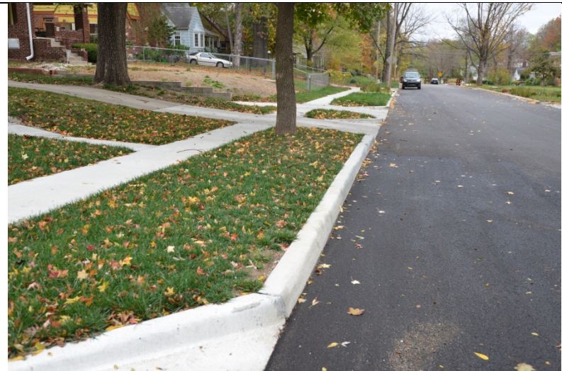
Upgradient from rain garden
