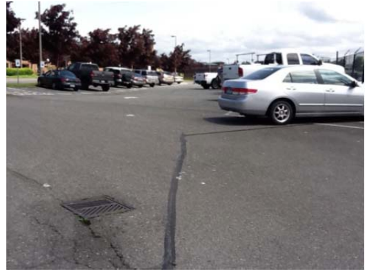
Paved parking area. Photo 24: Parking area north of Bldg. 2310.
