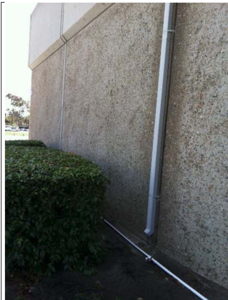
Photo 22: Bldg 698- Entire roof drains to pervious area- Mixed Use Area
