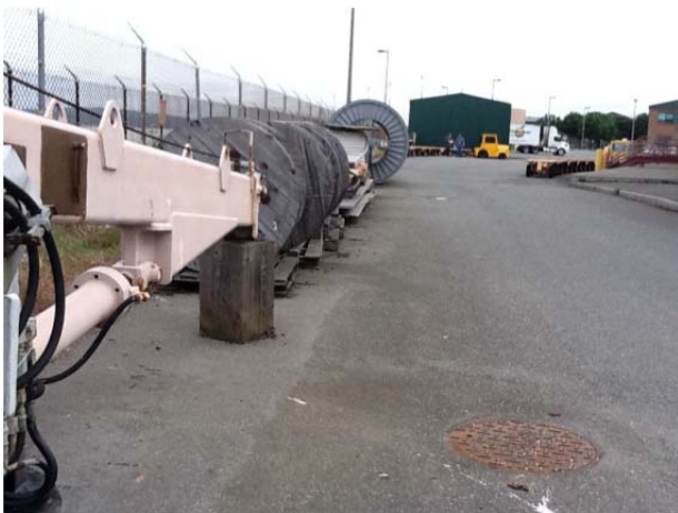
Asphalt, medium industrial storage/laydown area (other impervious area #7). Photo 5: Laydown area Bldg. 2200.
