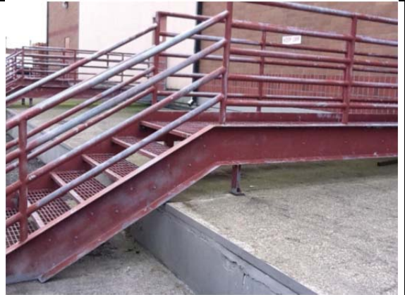
Other galvanized material area (other impervious area #10). Photo 15: Painted galvanized stairs/walkway rear of Bldg. 2202, note wear of paint.
