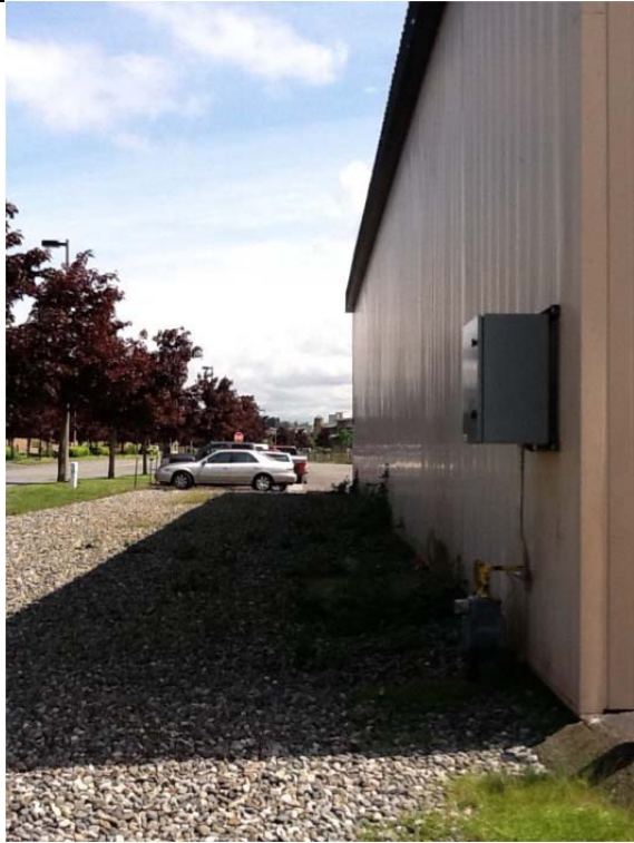
Roof drain to pervious area. Pervious rock landscape adjacent to Bldgs. 2320/2330/2310.
