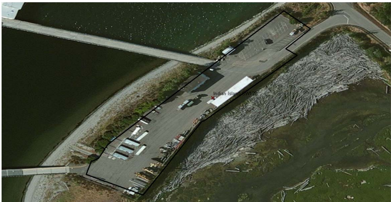
Watershed Boundary and Aerial Image for Naval Magazine Indian Island Outfall SW120
