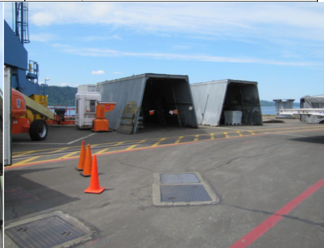
Galvanized metal roofs (other impervious area #9).Photo 11: Galvanized storage sheds, drains to ground.
