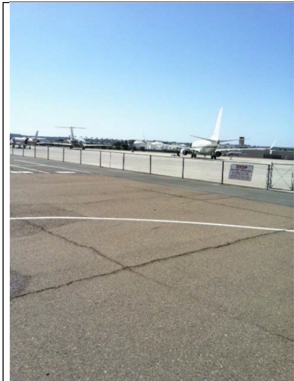
Photo 23: Asphalt lot- Airfield
