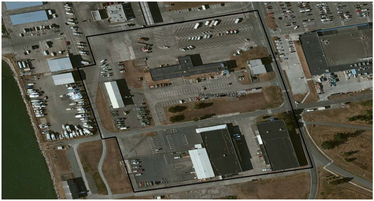
Watershed Boundary and Aerial Image for Whidbey Island Seaplane Base Outfall 3D
