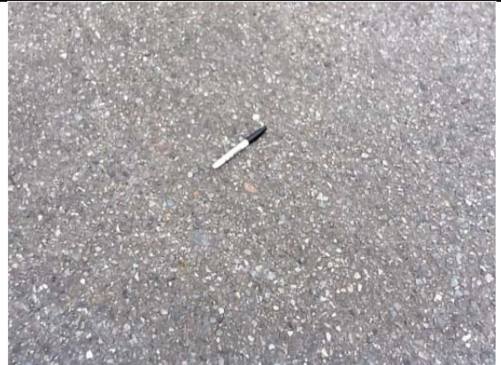
Paved parking area. Photo 11: Asphalt texture real Bldg. 2200.
