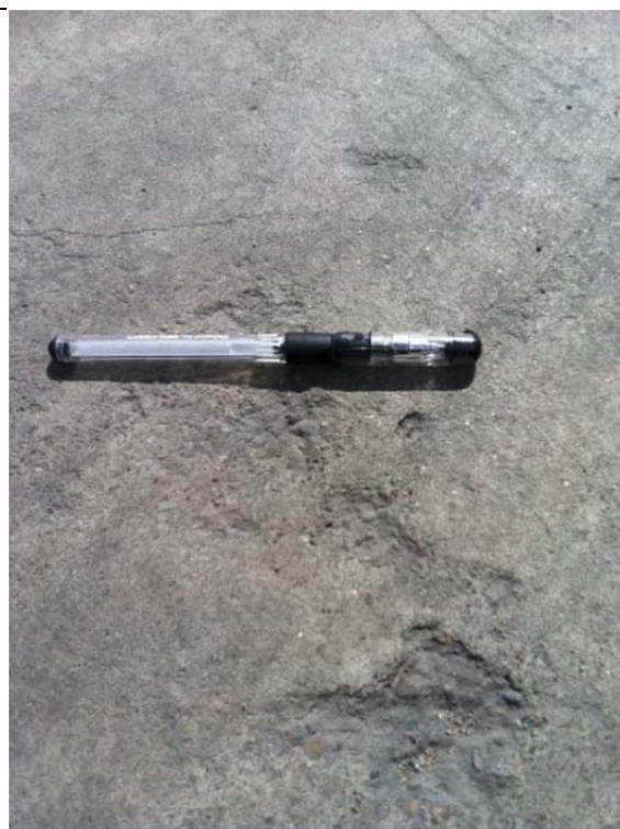
Photo 19: Concrete in good condition inside "concrete circle"- Industrial Southeast
