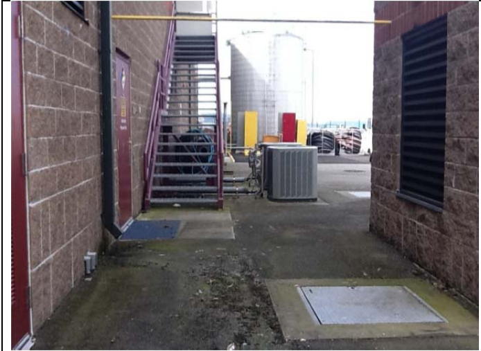
Other galvanized material area (other impervious area #10). Photo 14: Rear Bldg. 2300 showing painted galvanized stairway, drainage connection and misc. materials.
