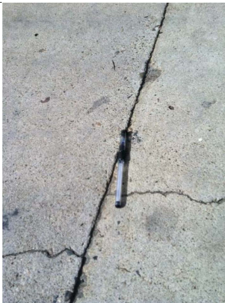
Photo 12: Concrete loading dock near bldg 789- Industrial West
