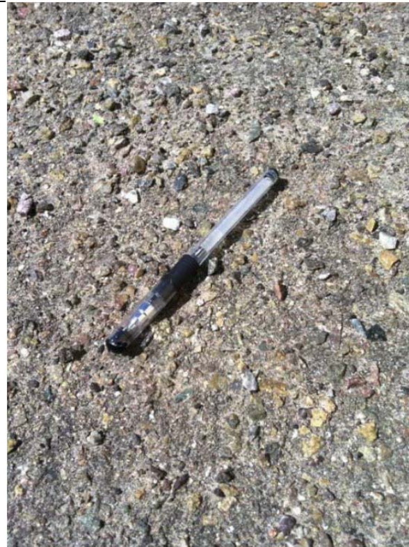
Photo 2: Rough Asphalt- Industrial North
