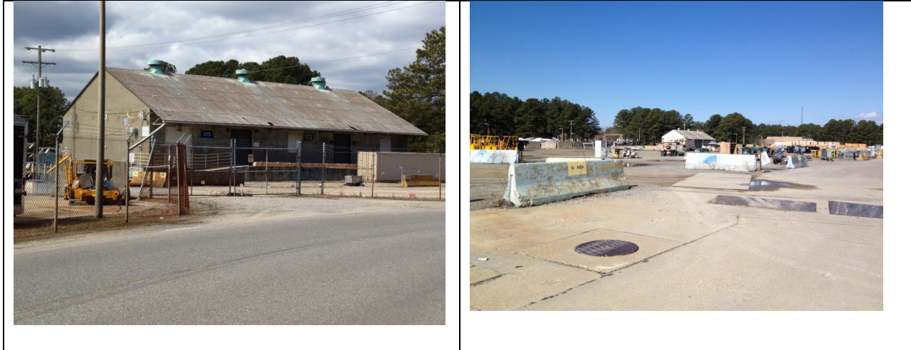
Photos taken during site surveys of St Juliennes OF 40 and 41
