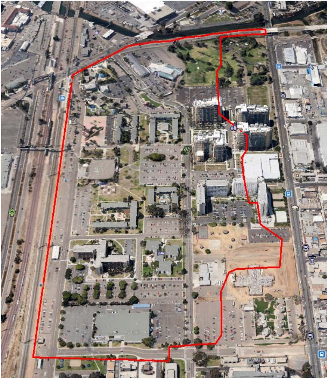
Aerial view and Outline of NBSD Outfall 70
