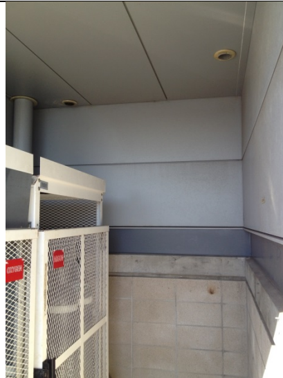
Bldg. 633 southwest corner roof drains
