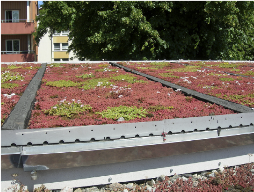
Fig.3 – Study site at the extensive vegetated roof at Augustenborg, Malmö, Sweden.
