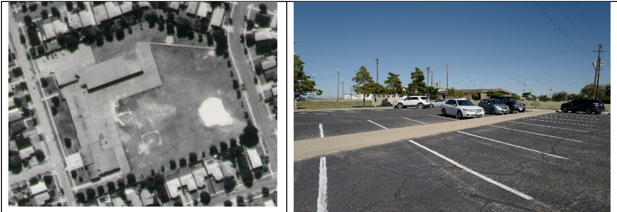
Institutional parking areas; small parking area for staff at elementary school and large parking area (with curbed dividers) for students at junior college.
