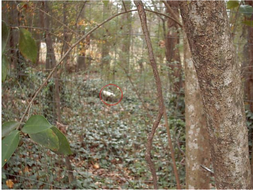
Figure 4.12. Pipe opening into ditch upstream to outfall 31
