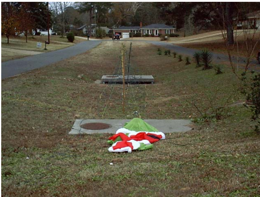
Figure 4.17. Residences Upstream to MH 39.1 and MH 39.2
