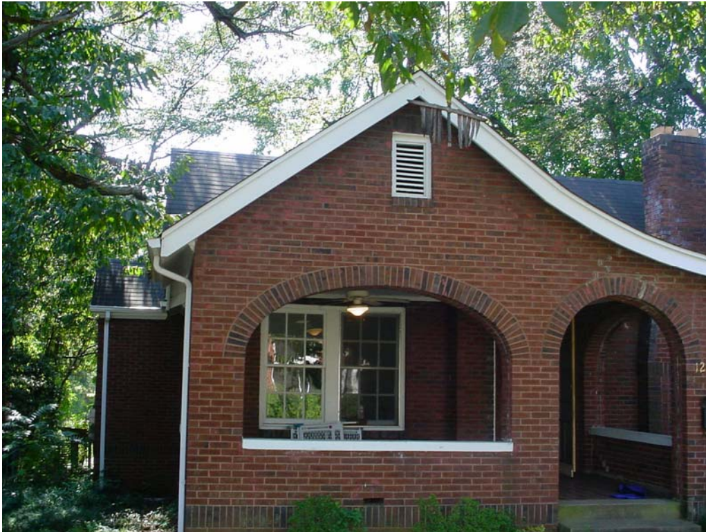
Figure 3.2 Roof with Canopy Cover (Roof – P)
