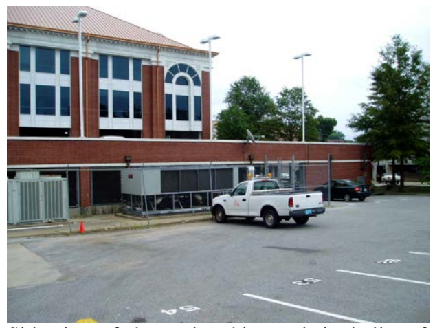
Side view of elevated parking and city hall roof and drains to test area.
