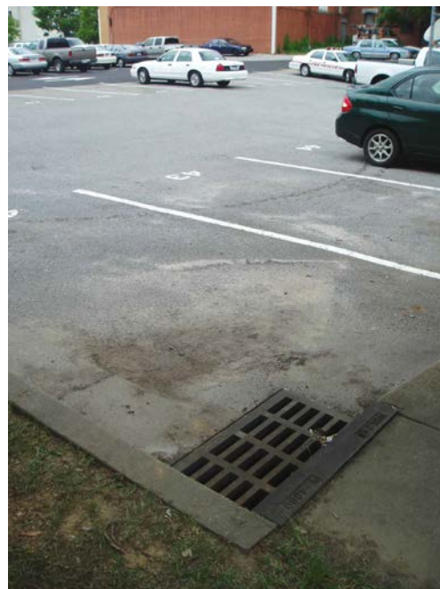
About 1/4 acre of asphalt paved parking area draining to inlet.
