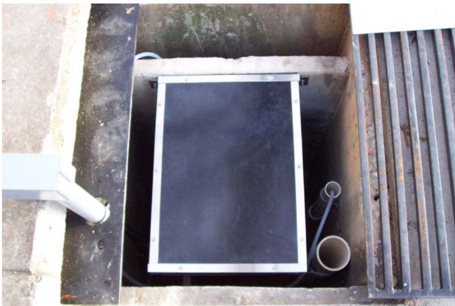
Figure 4.10: Prototype UpFlow™ filter with cover installed.
