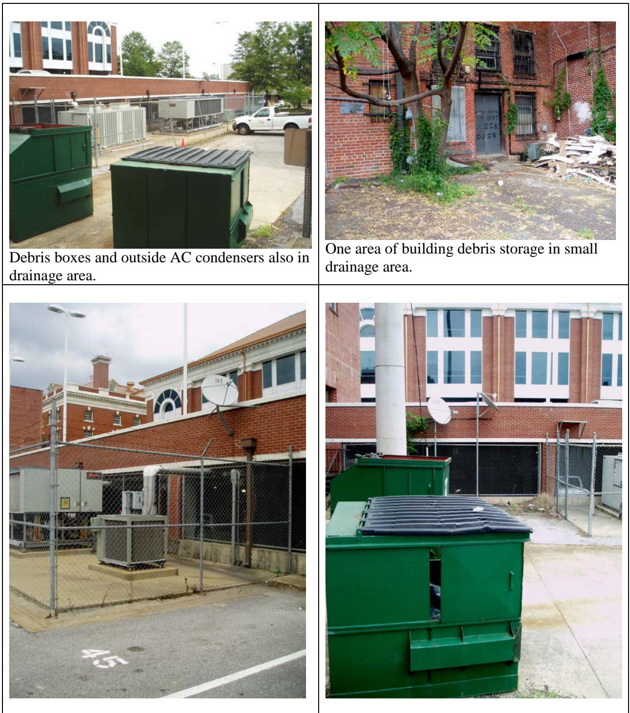
Figure 4.17: Views of test area drainage.
