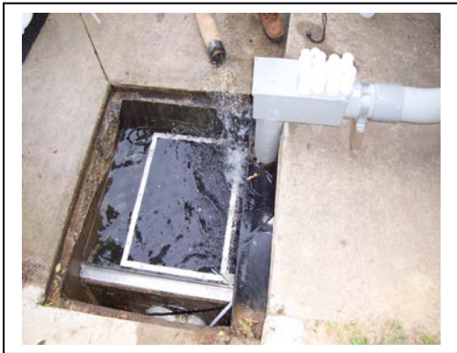
Figure 5.13: Flow right at the overflow
