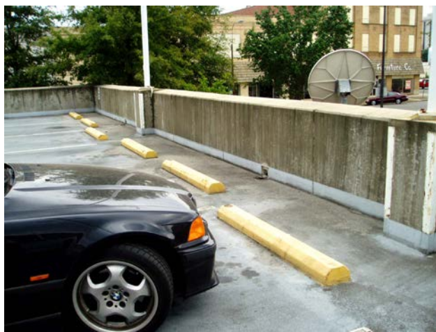
Elevated concrete parking area that also drains to test area.
