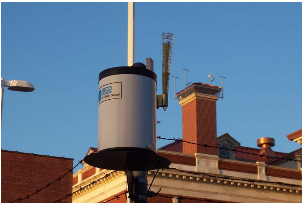
Figure 4.14: Tipping bucket and standard rain gauges installed at monitoring site.
