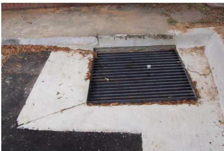
Figure 4.11: Completed modified inlet with new inlet grating.
