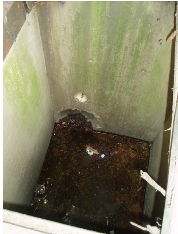
15 inch outlet in bottom corner (small 4 inch outlet above, from landscaped area)
