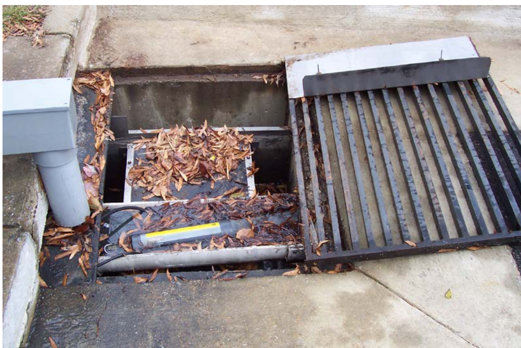
Figure 6.4: Picture showing the influent sample tray and the sonde.
