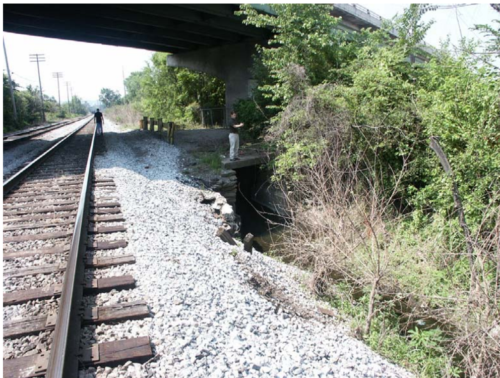
Fig. B4. Outfall 001 Surrounding Area
