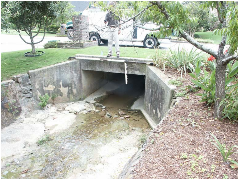
Fig. B17. Outfall 010 General View
