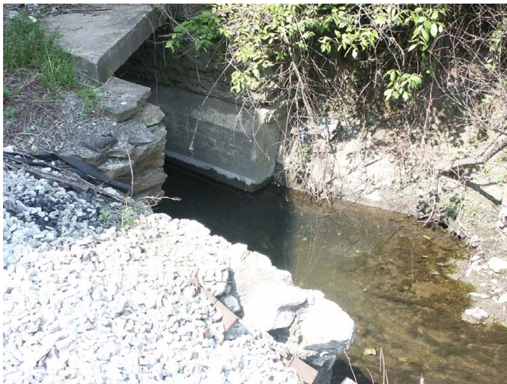
Fig. B5. Outfall 001 General View
