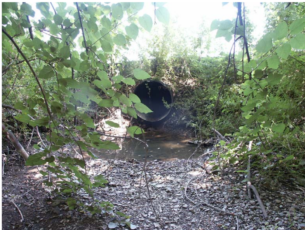
Fig. B9. Outfall 002 General View
