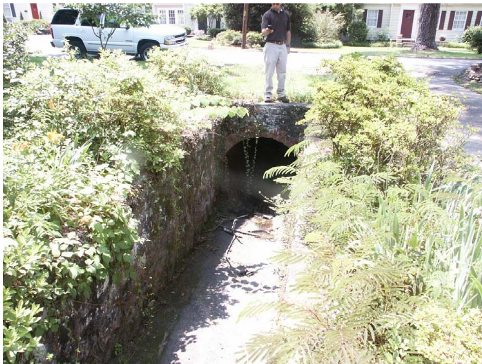
Fig. B13. Outfall 009 General View
