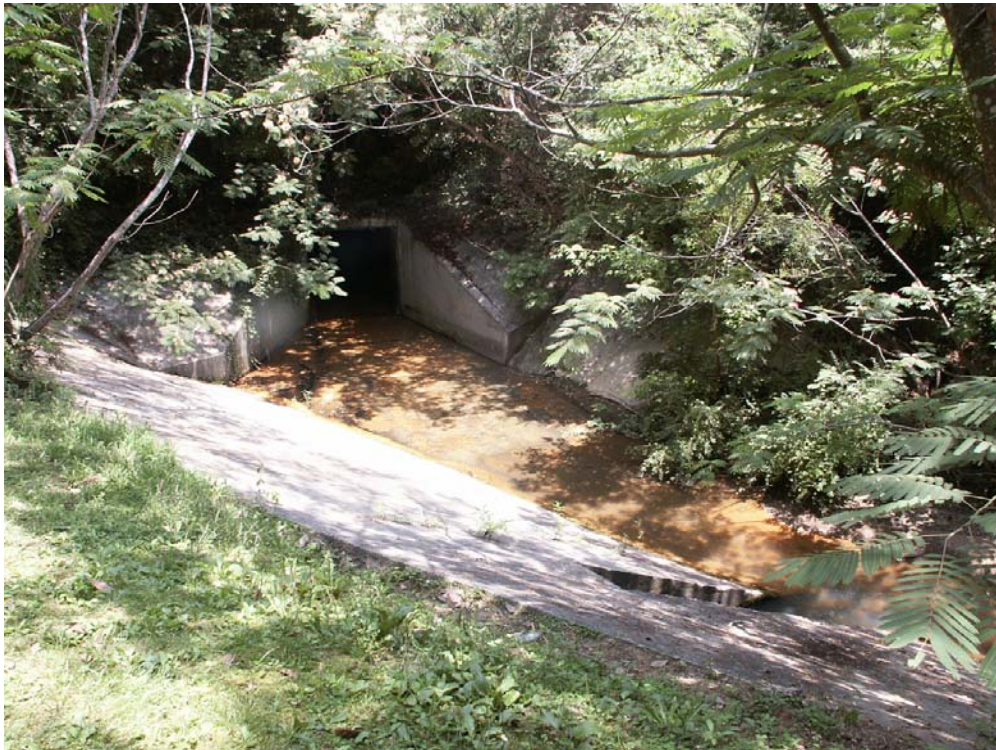
Fig. B 21. Outfall 012 General View
