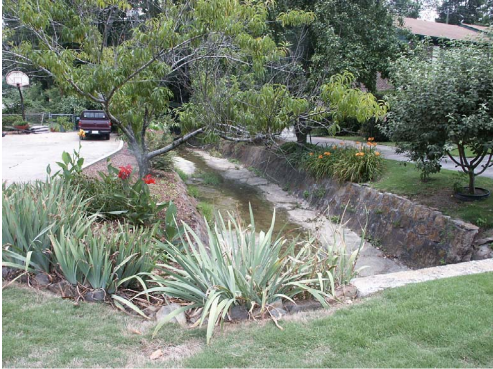
Fig. B16. Outfall 010 Surrounding Area
