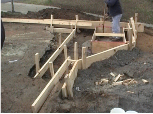
Filter inlet formwork
