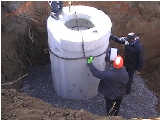
Filter placement in cut
