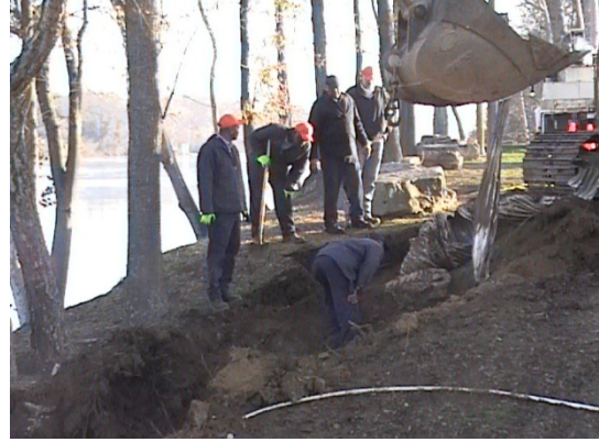
Removal of old inlet and excavation
