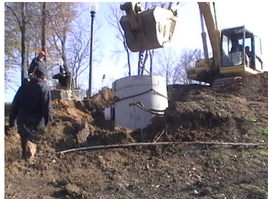
Hoisting filter into cut
