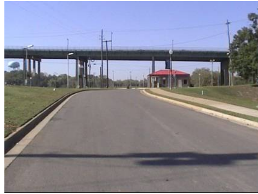
Sidewalks and roadway to the parking lot
