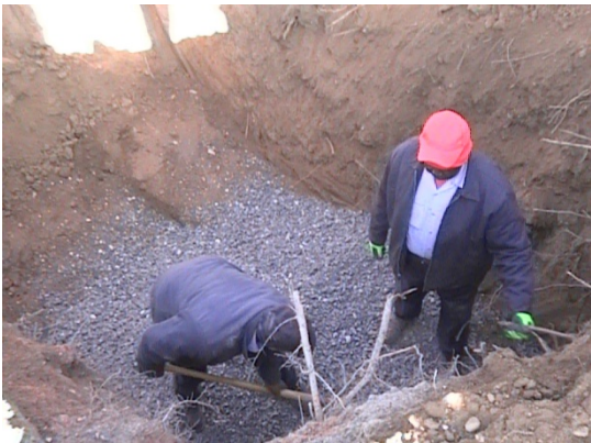
Gravel to level elevation
