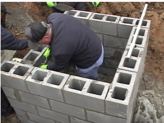
Effluent sampling box installation
