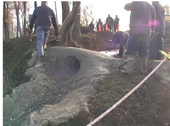
Outfall to Black Warrior River
