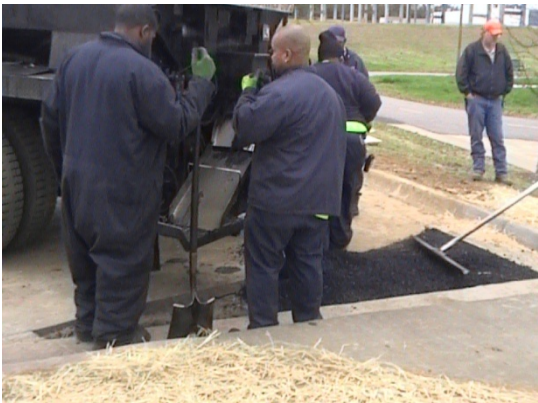
Asphalt repair
