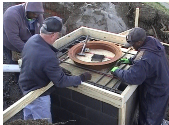
Top of the sampling box construction
