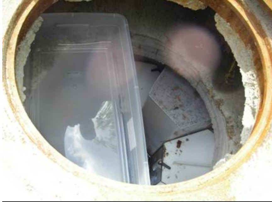
Figure 28. Influent Sample is Collected in the Sample Tray
