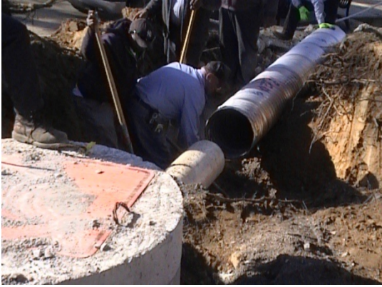
Backfilled and connecting outlet pipe
