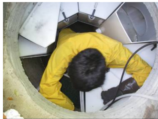
Media is installed with green base
