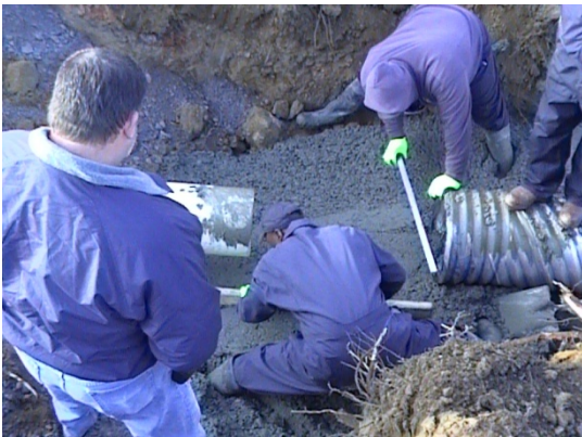
Leveling floor of effluent chamber
