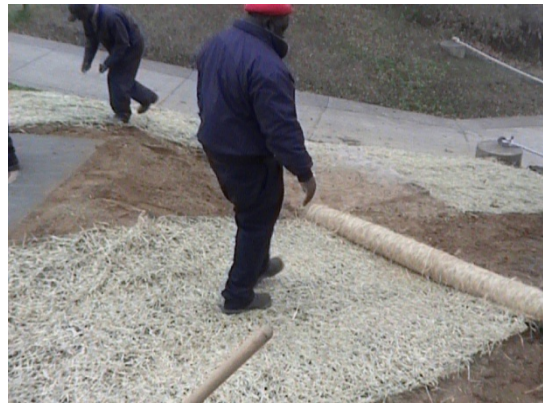
Seeding and erosion control
