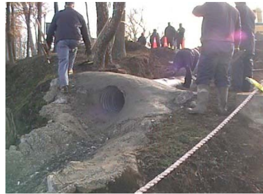
Outfall to Black Warrior River
