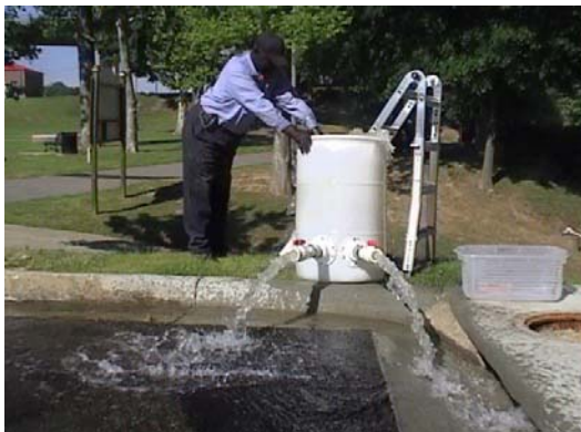
River water is pumped into the plastic flow splitter barrel
