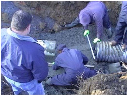
Leveling floor of effluent chamber
