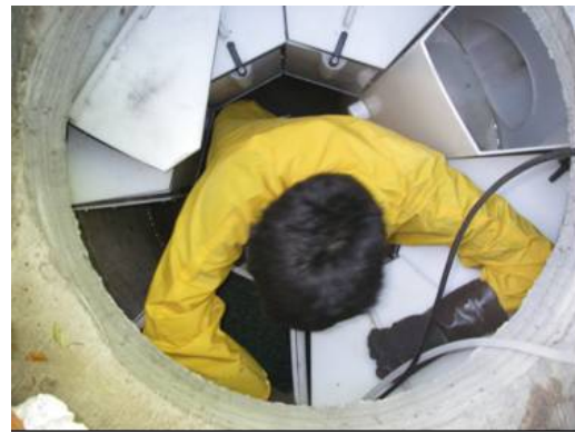
Media is installed with green base
