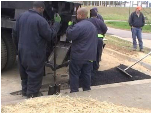
Asphalt repair
