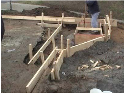
Filter inlet formwork
