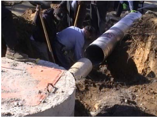
Backfilled and connecting outlet pipe
