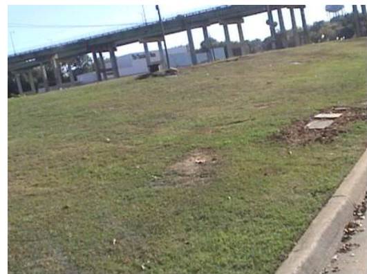
Turf area on the side of the road
