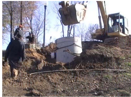
Hoisting filter into cut
