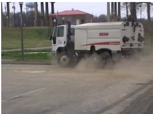
Final site clearing
