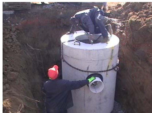
Checking the level and elevation of the filter
