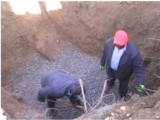
Gravel to level elevation
