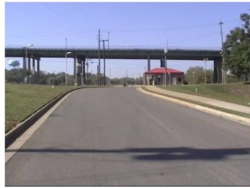
Sidewalks and roadway to the parking lot
