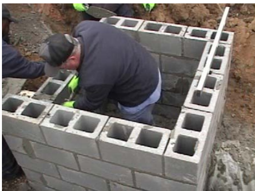
Effluent sampling box installation
