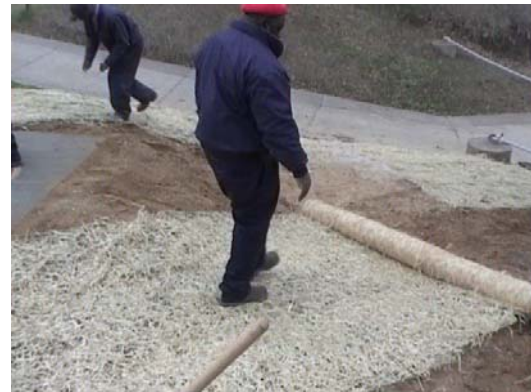
Seeding and erosion control
