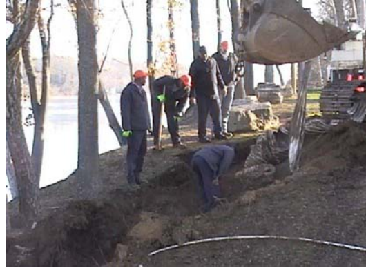
Removal of old inlet and excavation
