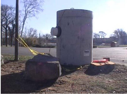
Filter before the installation
