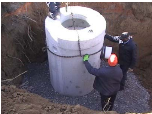
Filter placement in cut
