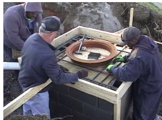
Top of the sampling box construction
