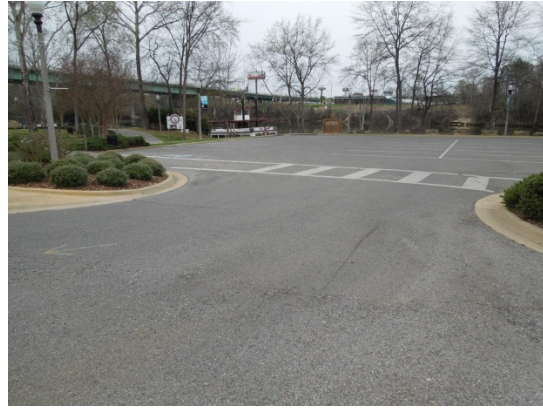
Large fraction of impervious asphalt pavement and crosswalk
