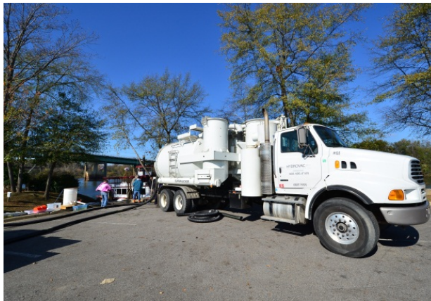
Vacuum truck used to clean out Up-Flo ® Filter vault
