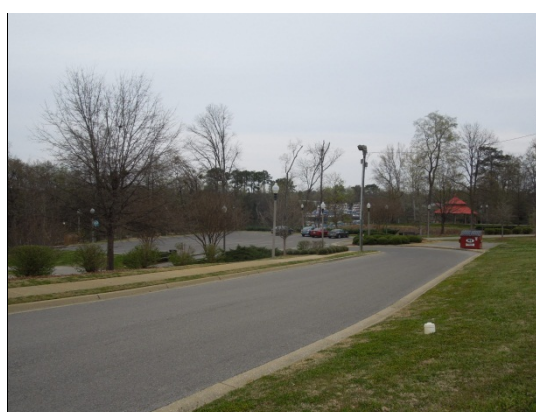
Slight slope in the parking entrance road directs the runoff into the parking area
