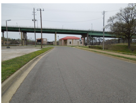
Only one building at the site with small roof area
