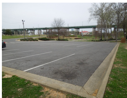
Asphalt pavement with apparent vehicle oil and grease on the surface
