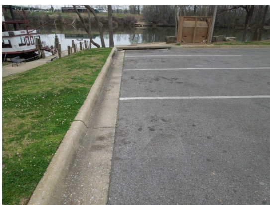
Runoff enters filter inlet through roadside gutter and sheet flow
