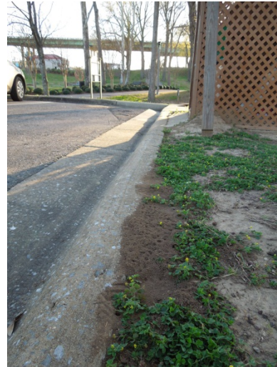
Ant hills beside the filter inlet may affect the influent quality during storms
