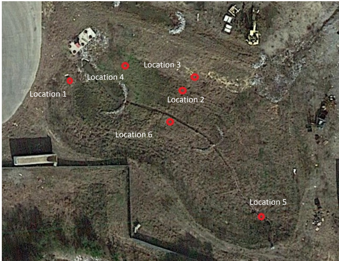
Figure 3-42 Dry pond infiltration test locations
