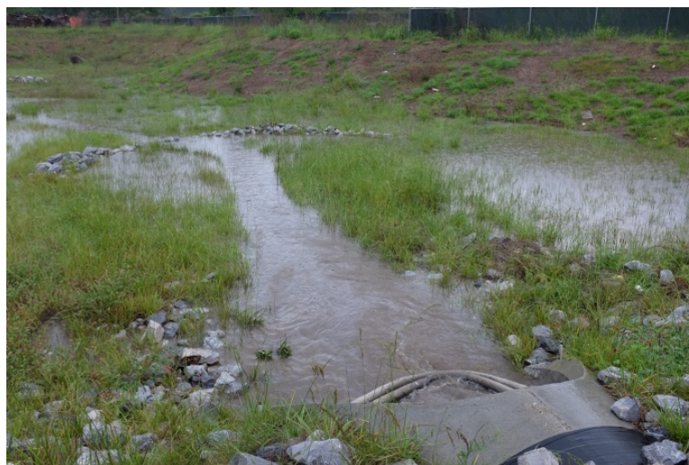
Figure 4-2 Dry pond after period of very intense rain showing partial flooding of pond
