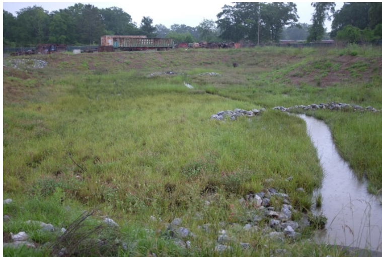
Figure 4-1 Dry pond with rock check dams showing channel and grass cover
